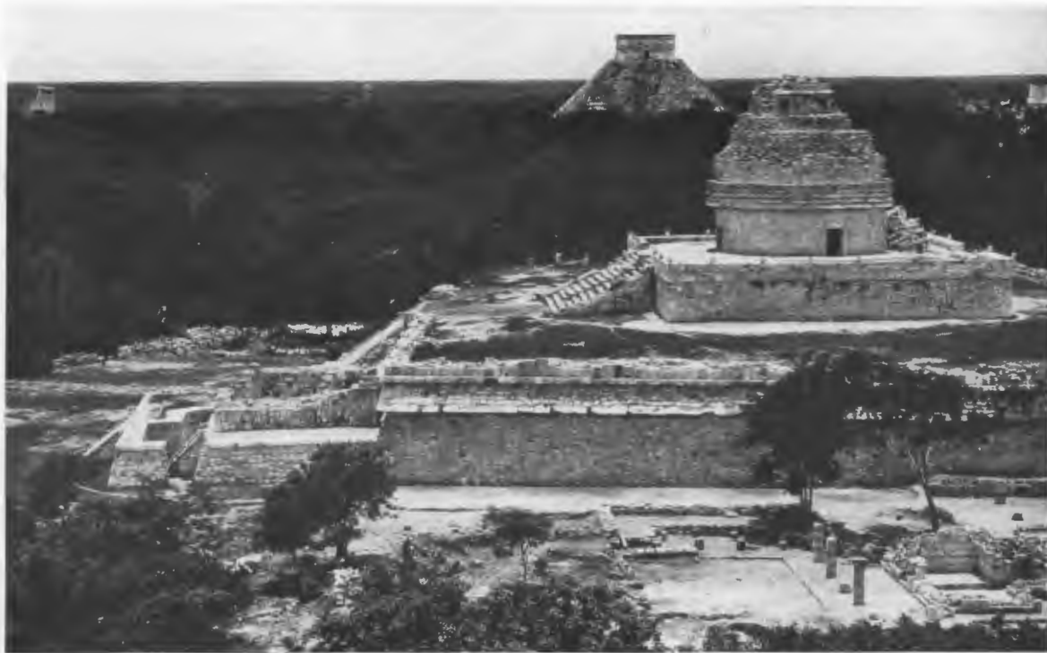
FIG. 20—SOUTHWEST CORNER OF LOWER PLATFORM AFTER REPAIR WAS COMPLETED.
