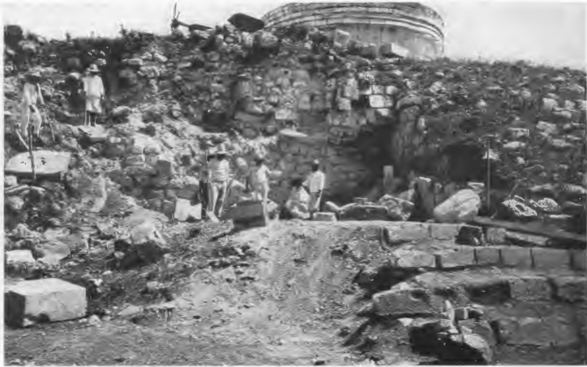
FIG. 27—LOWER PLATFORM NORTH OF STAIRWAY, BEFORE REPAIR.
