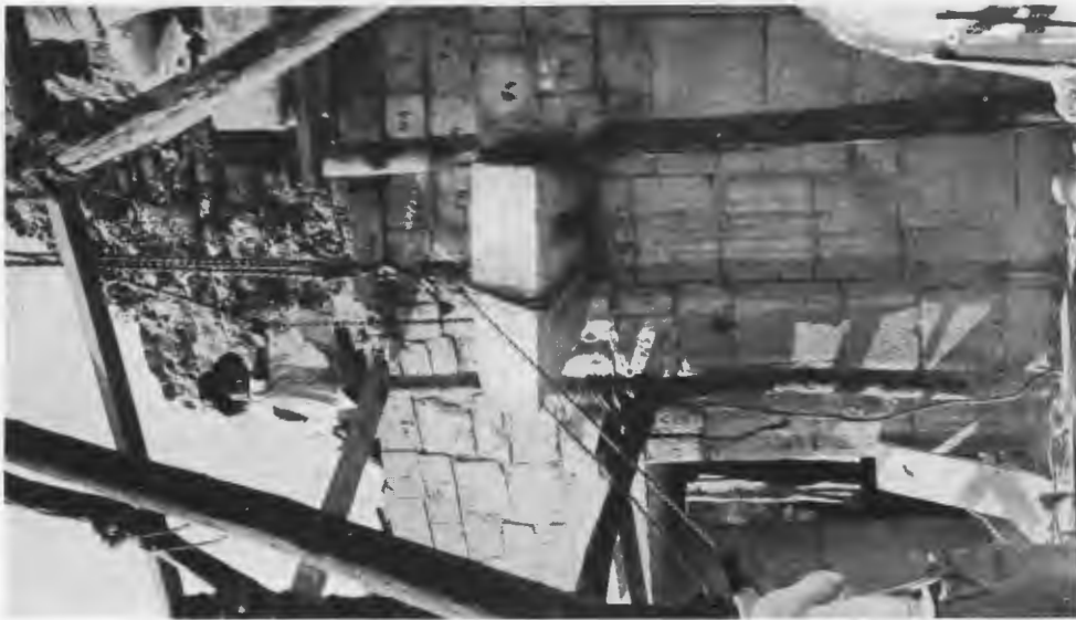
FIG. 214.—Raising stone by means of chain block.
