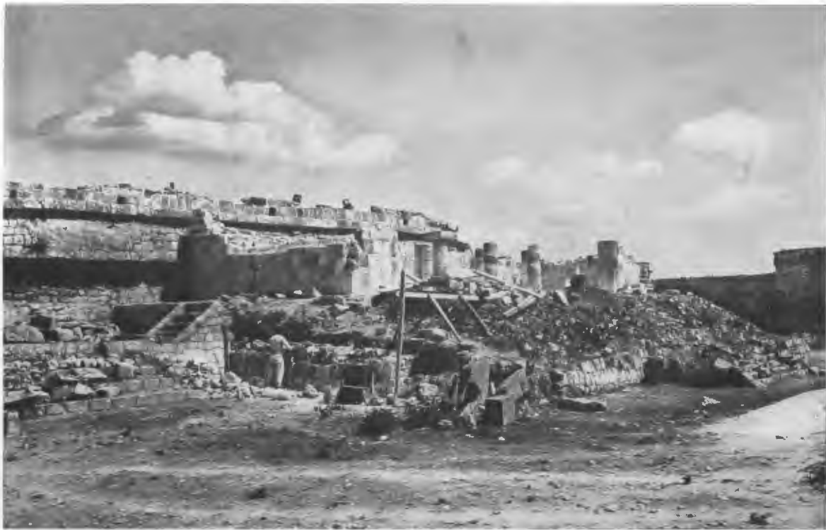
FIG. 309—CARACOL WEST ANNEX, SEEN FROM NORTHWEST AFTER EXCAVATIONS WERE COMPLETED. MASON IS REPAIRING PLATFORM FACING.
