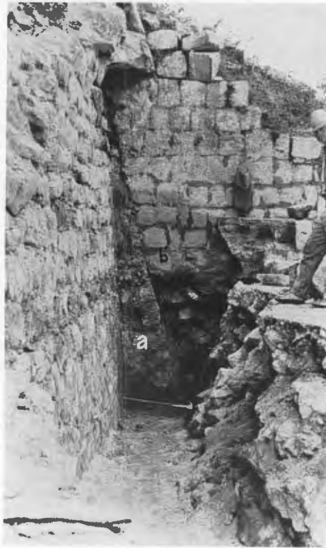
FIG. 56—EXCAVATIONS FOR STUDY OF LOWER PLATFORM STAIRWAY, NORTH SIDE.
