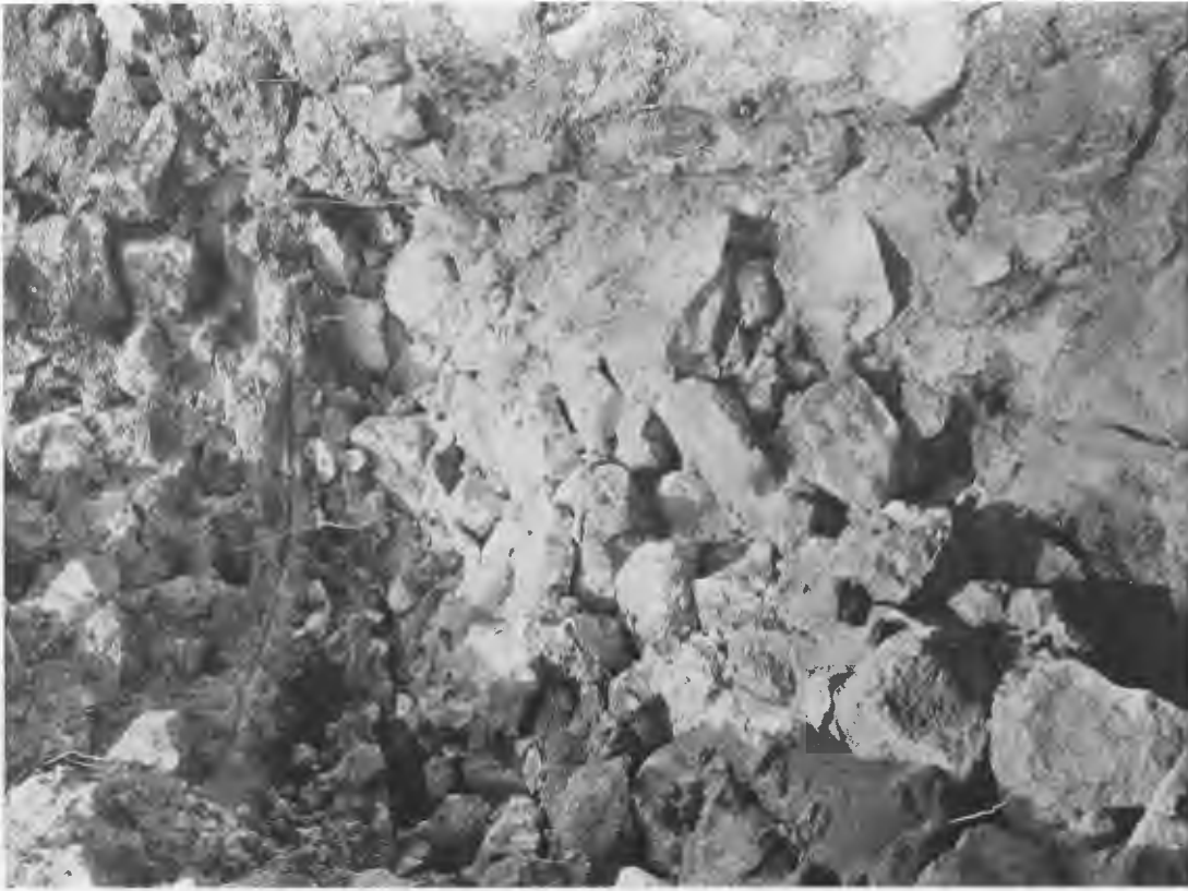
FIG. 71—FILL BEHIND STAIRWAY OF LOWER PLATFORM SOLIDLY PACKED.
