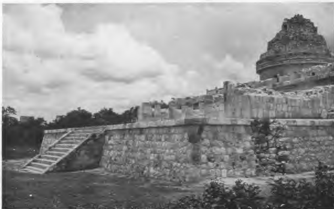
FIG. 301—CARACOL WEST ANNEX, REPAIR COMPLETED. View from southwest. Break in facing of south side of platform gives access to passageway across west face of early platform.
