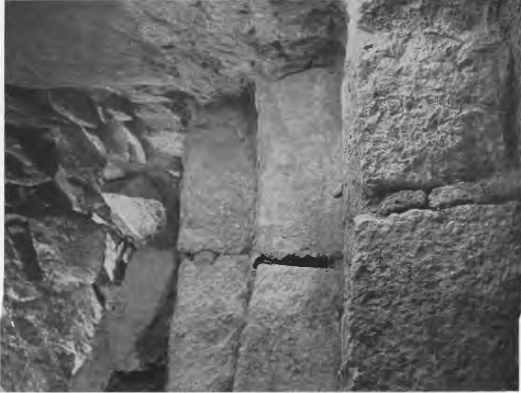
FIG. 286—SPIRAL STAIRWAY IN MASONRY CORE, NOT REPAIRED.
