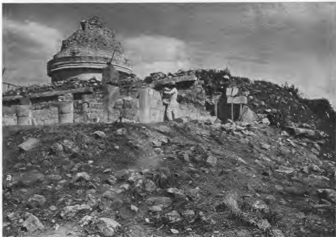
FIG. 328—CARACOL WEST ANNEX, VIEWED FROM SOUTHWEST BEFORE PLATFORM WAS EXCAVATED.
