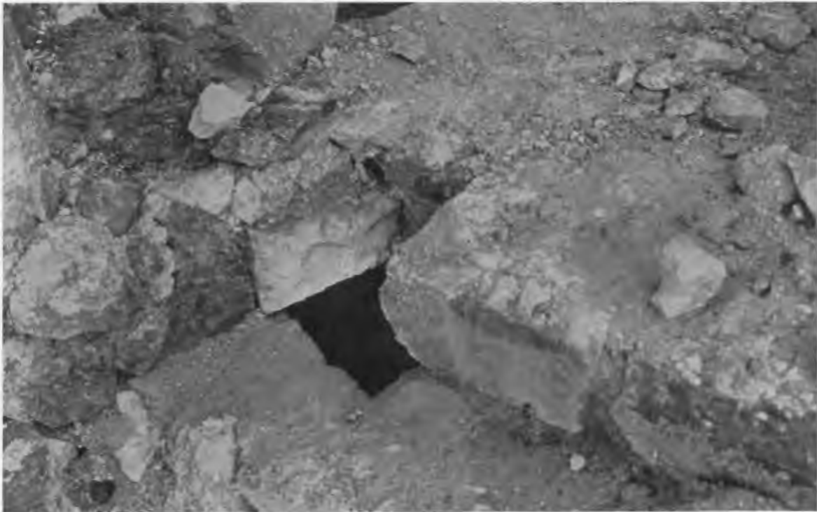
FIG. 154—ORIFICE OF A WEEP HOLE IN NEXT TO LAST RISER OF STAIRWAY AND ON SOUTH SIDE OF MASONRY BLOCK WHICH DIVIDES UPPER SECTION OF STAIRWAY.
