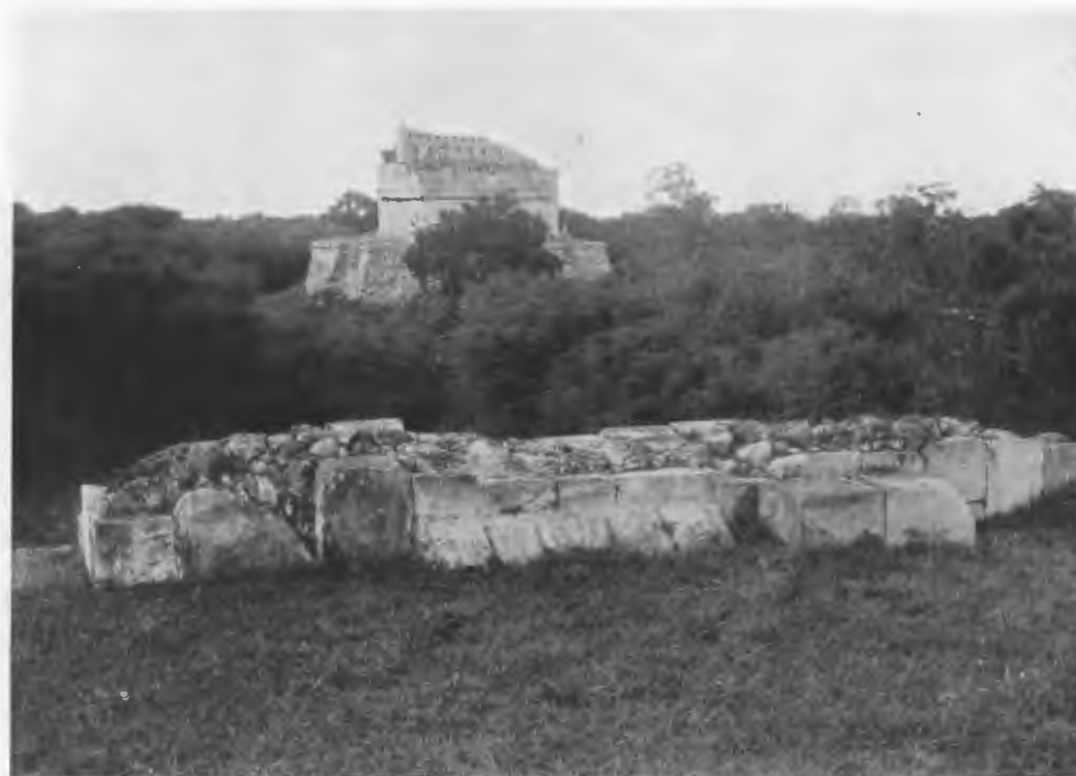
FIG. 18—PARAPET OF LOWER PLATFORM, NORTH OF STAIRWAY, REPAIRED.
