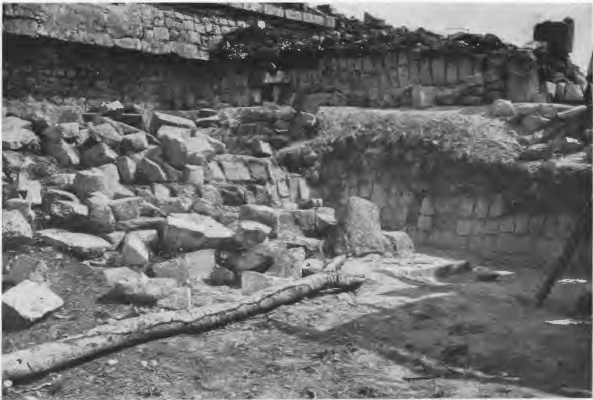
FIG. 300—CARACOL WEST ANNEX, LATE PLATFORM, NORTH SIDE. Masonry facing is of dressed stones applied as veneer.
