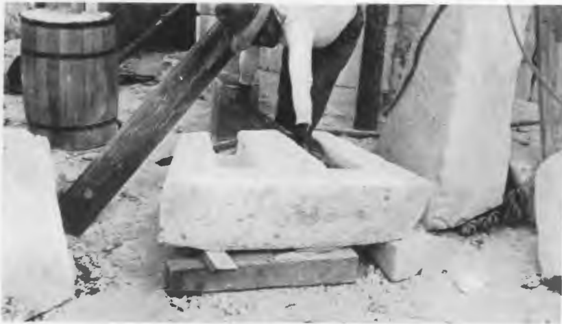
FIGS. 211, 212 AND 213—CARACOL TOWER, REPAIR OF FIVE-MEMBER MOLDING.
