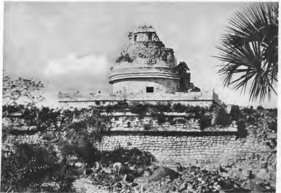
FIG. 244—CARACOL TOWER, SOUTH SIDE, REPAIR COMPLETED IN 1930.
