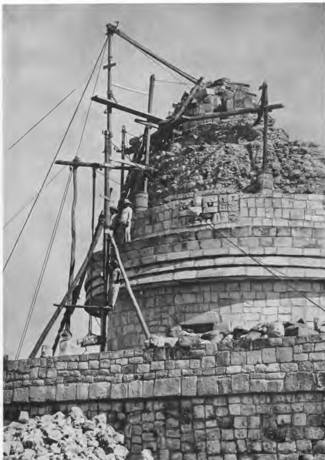
FIG. 242—CARACOL TOWER DURING REPAIR IN 1930.
