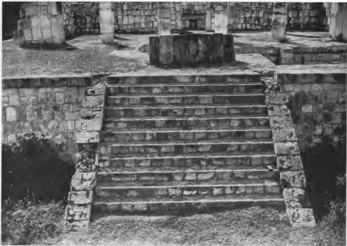
FIG. 307—West stairway repaired. Each balustrade bears a low-relief carving of a plumed serpent.
