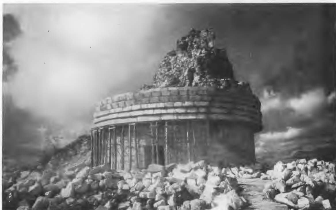
FIG. 205—PORTION OF FIVE-MEMBER MOLDING OF NORTH SIDE REPAIRED IN 1927.
