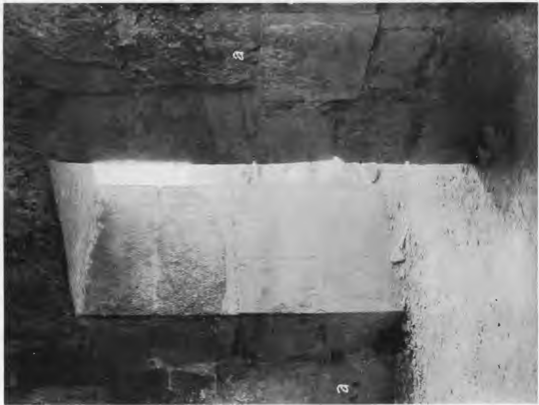
FIG. 187—VIEW IN OUTER ANNULAR CHAMBER OF TOWER. West doorway. Cord-holders, a , were placed at either side of all doorways.
