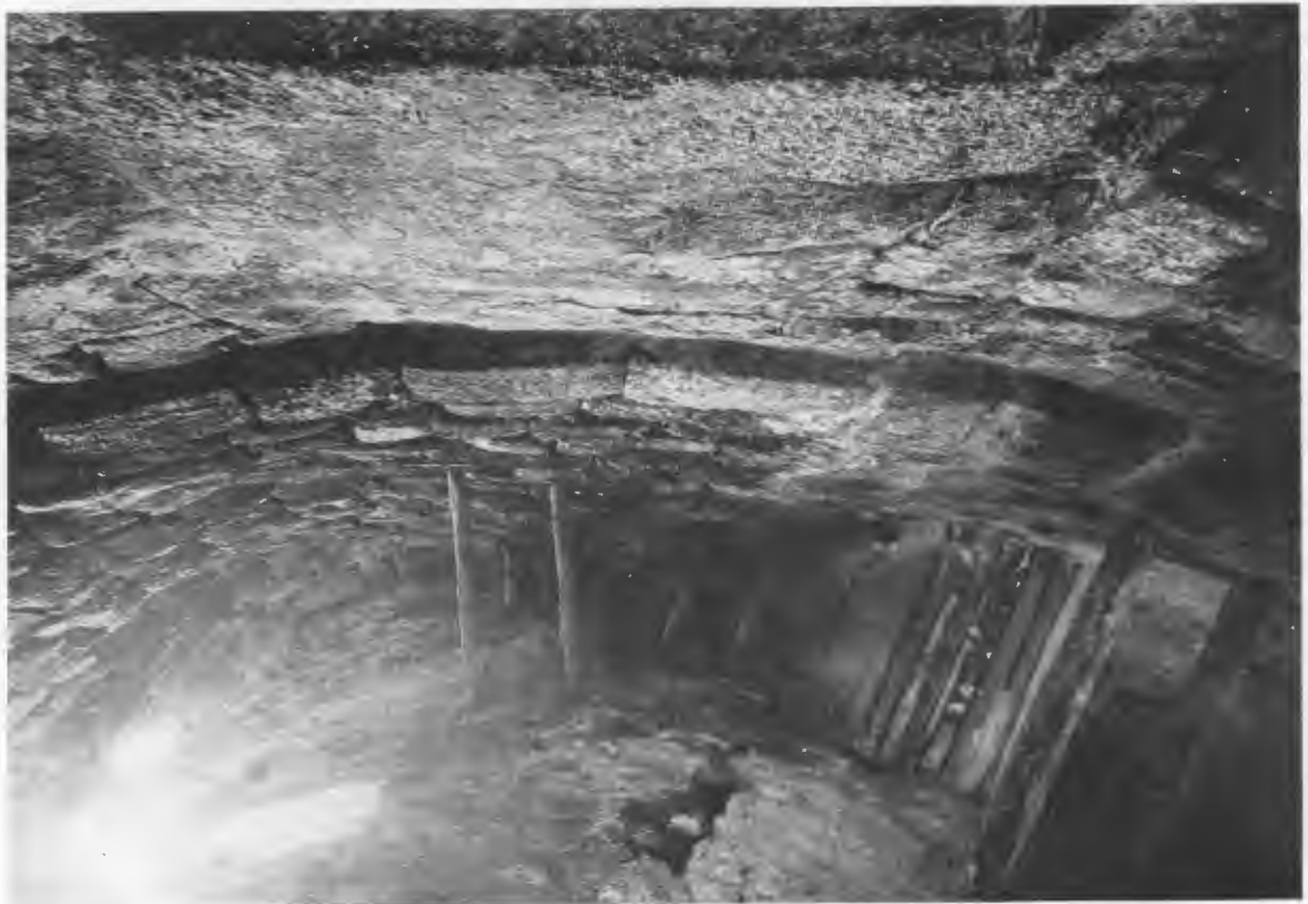
FIG. 268—VIEW LOOKING UPWARD INTO ARCH OF OUTER ANNULAR CHAMBER, WEST QUADRANT.
