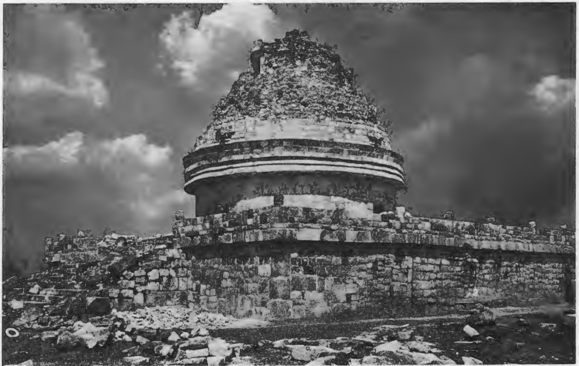
FIG. 136—UPPER PLATFORM, SOUTH SIDE. REPAIR COMPLETED IN 1929.
