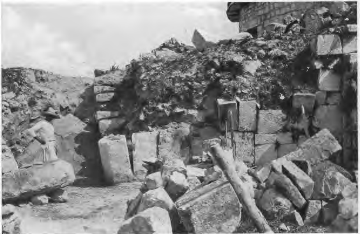
FIG. 132—EXCAVATION OF NORTHWEST CORNER OF UPPER PLATFORM.
