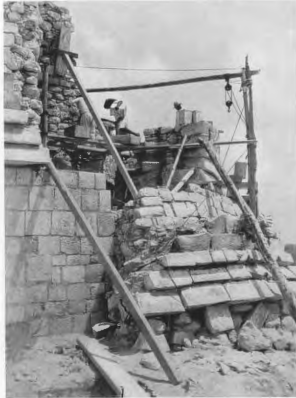
FIG. 199—BLOCK OF FALLEN MOLDING WITH SECTION OF UPPER VERTICAL ZONE.
