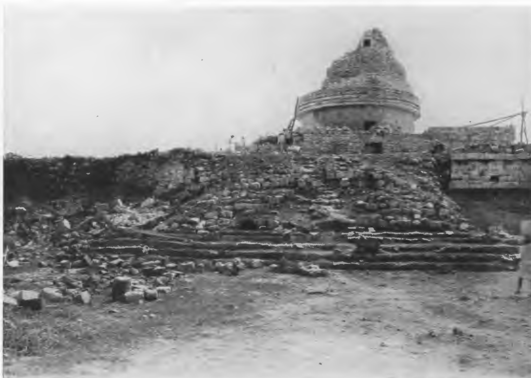
FIG. 73—LOWER PLATFORM STAIRWAY BEFORE REPAIR.
