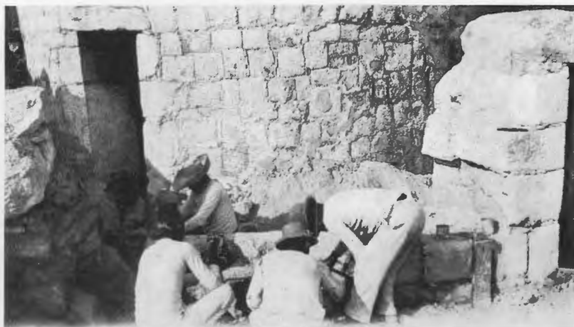
FIG. 271—REPAIR OF OUTER WALL OF TOWER.
