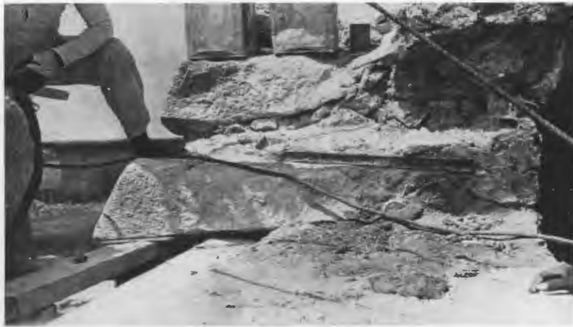
FIG. 216—REPAIR OF FIVE-MEMBER MOLDING.
