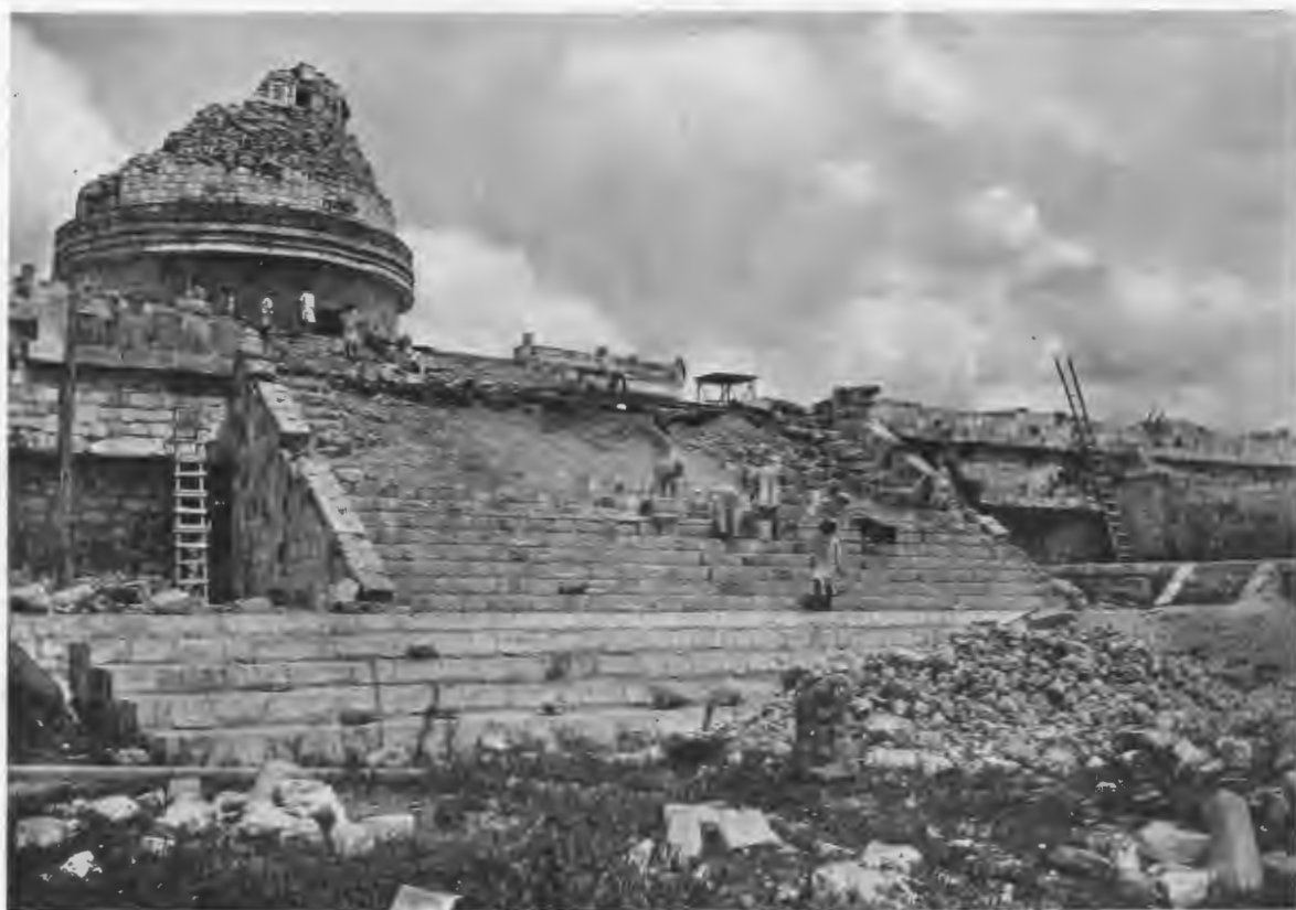
FIGS. 88 AND 89—REPAIRING LOWER PLATFORM STAIRWAY.
