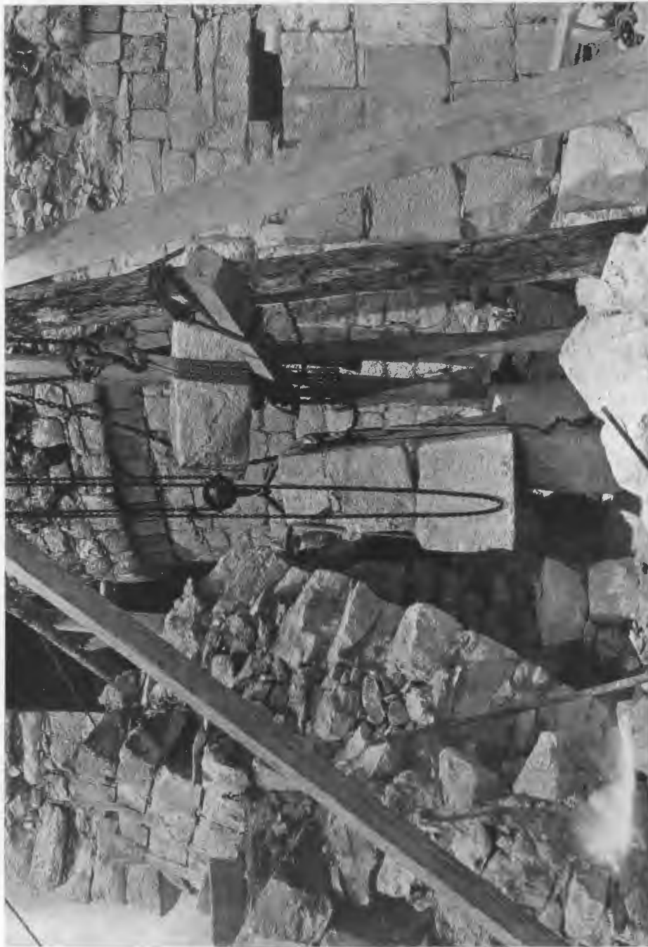
FIG. 252—CARACOL TOWER, REPAIR OF EAST DOORWAY.
