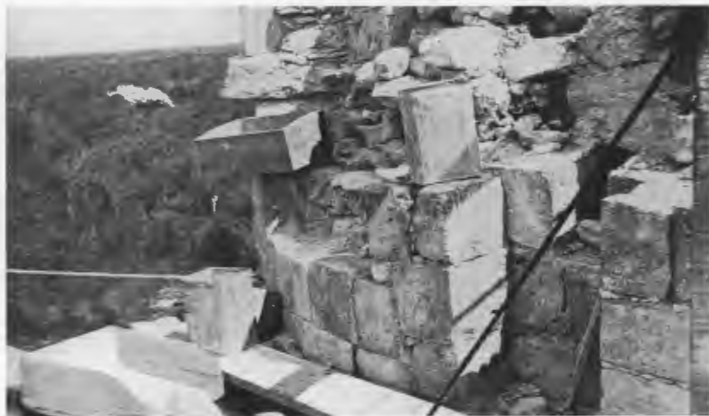
FIG. 241—CARACOL TOWER, REPAIR OF SOUTHWEST RECESS OF UPPER STORY.
