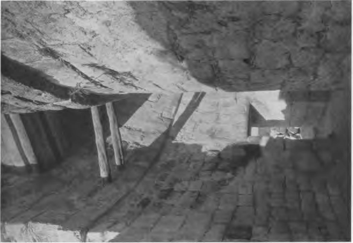
FIG. 256—CARACOL TOWER, OUTER ANNULAR CHAMBER. SOUTH DOORWAY.
