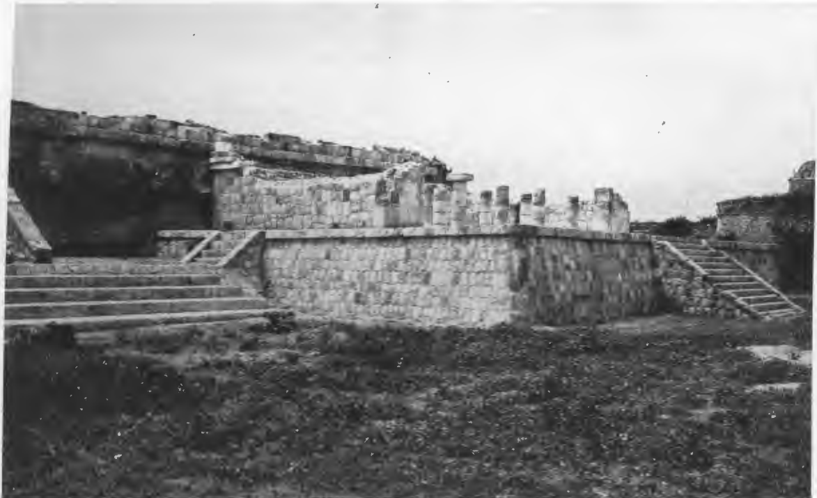
FIG. 310—CARACOL WEST ANNEX, SEEN FROM NORTHWEST, AFTER REPAIR WAS COMPLETED. PHOTOGRAPH TAKEN IN 1929.
