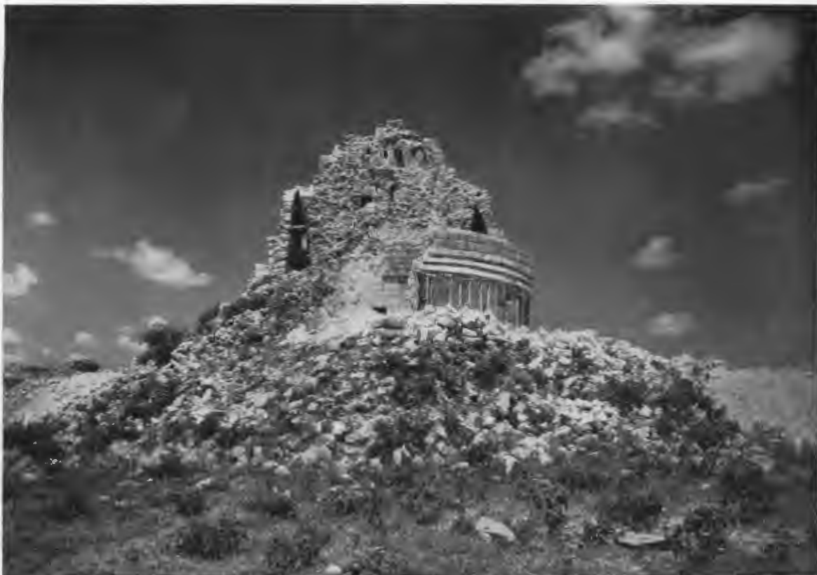
FIG. 137—NORTHEAST CORNER, UPPER PLATFORM, BEFORE EXCAVATION IN 1927.
