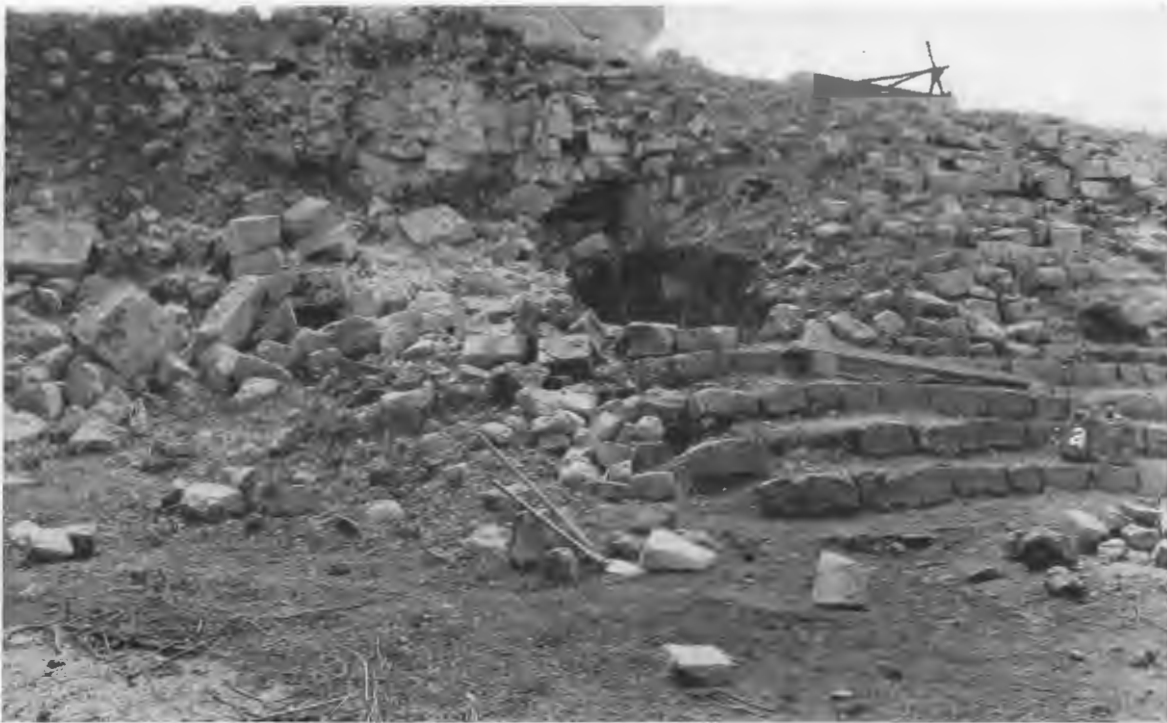
FIG. 75—LOWER STAIRWAY, NORTH SIDE.
