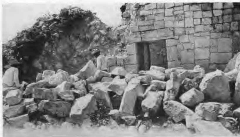
FIG. 189—MASONRY, NORTH DOORWAY OF TOWER.
