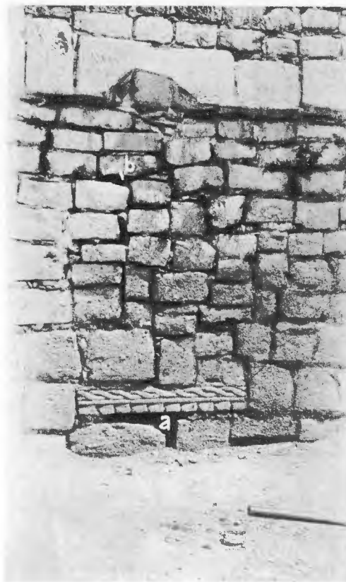
FIG. 153—SCULPTURED STONE REUSED IN SOUTH FACING OF EASTERN EXTENSION OF RECTANGULAR PLATFORM.
