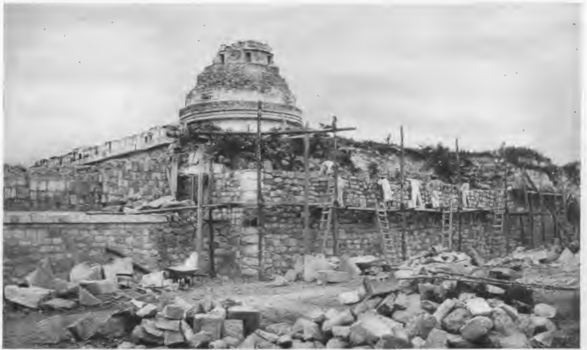
FIG. 21—LOWER PLATFORM, SOUTHWEST CORNER. REPAIRING LOWER ZONE.
