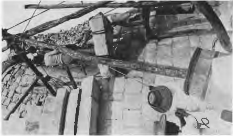
FIG. 210—RAISED TO PROPER HEIGHT, A SECOND CHAIN BLOCK WAS OFTEN NEEDED TO SWING STONE INTO POSITION.
