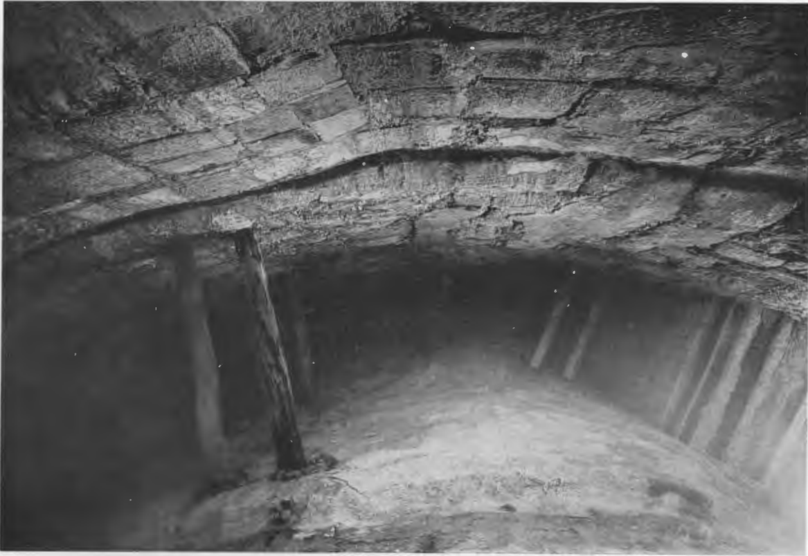
FIG. 269—VIEW LOOKING UPWARD INTO ARCH OF OUTER ANNULAR CHAMBER, SOUTH QUADRANT.
