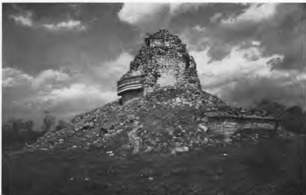
FIG. 133—SOUTHWEST CORNER OF UPPER PLATFORM. Photograph taken in 1925 before excavation.
