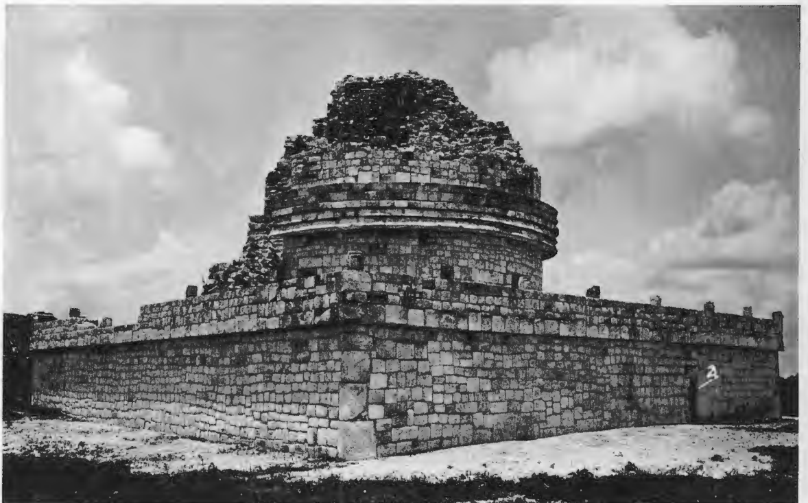
FIG. 140—NORTHEAST CORNER OF UPPER PLATFORM AND TOWER. View taken in 1930 after uprights had been removed from beneath five-member molding and platform cleared of débris. a , opening left in facing of platform to give access to trench exposing north side of second circular platform.
