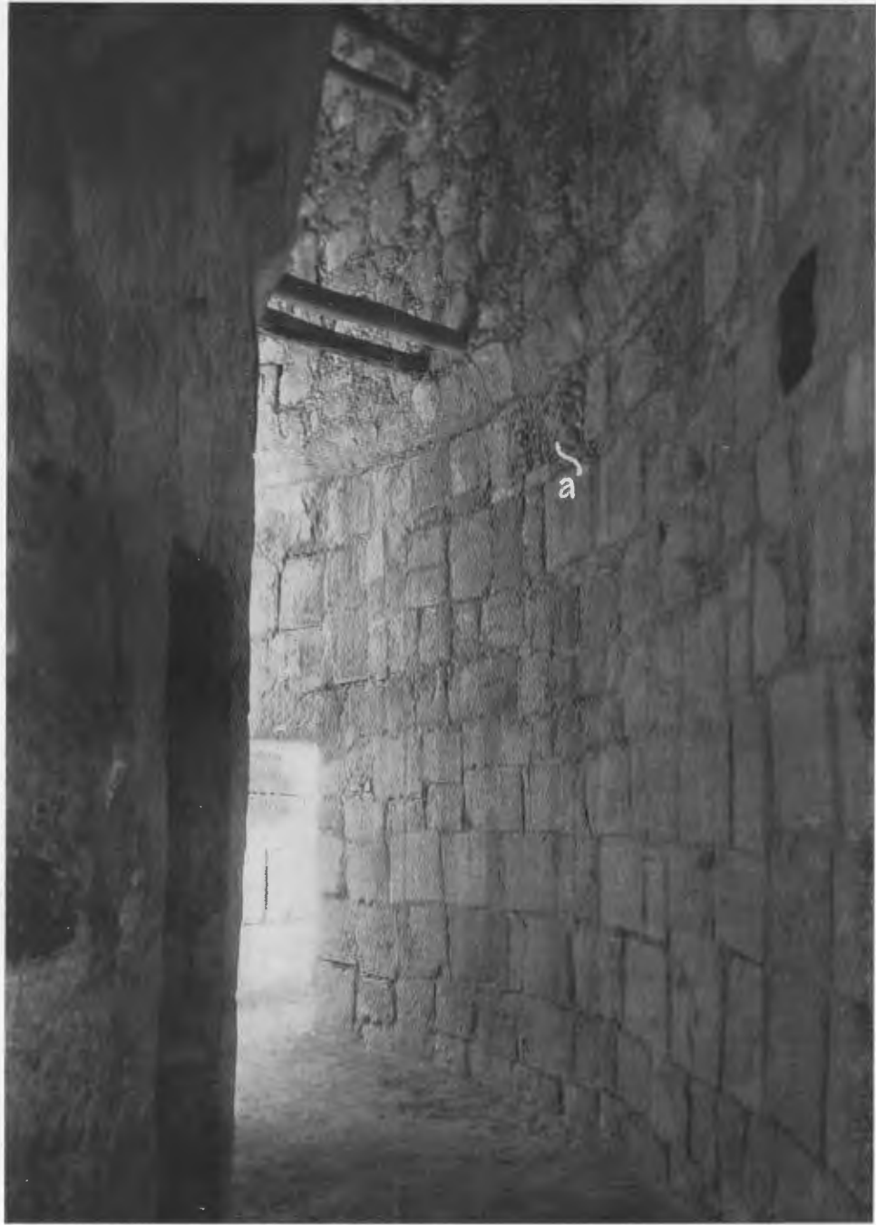
FIG. 194—CARACOL TOWER. SOUTHWEST QUADRANT OF OUTER ANNULAR CHAMBER. Butt of tenon, a , of first member of five-member molding forms facing stone in chamber.
