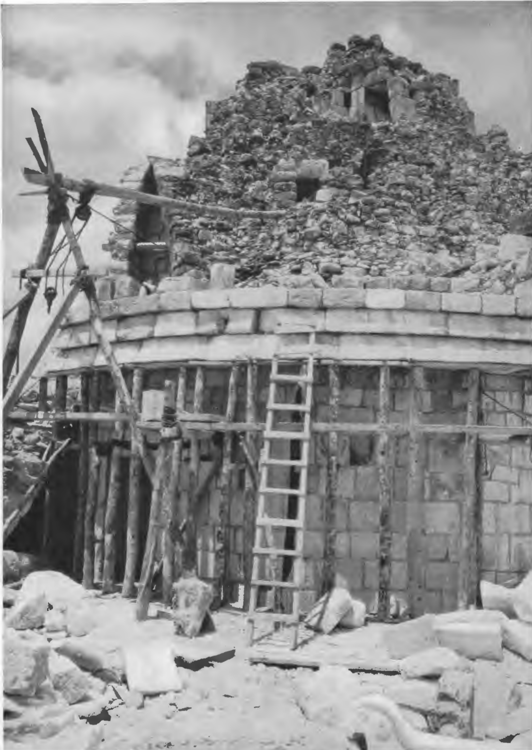
FIG. 207—CARACOL TOWER, NORTH SIDE, REPAIR OF FIVE-MEMBER MOLDING. Wooden uprights were used to help support molding while being replaced and until cement mortar had set.
