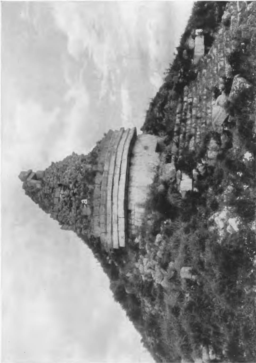
FIG. 219—CARACOL TOWER. Three courses of vertical zone, a , above five-member molding were found in situ .
