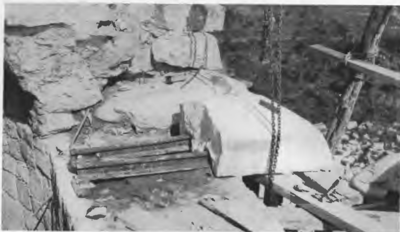
FIG. 218—STEEL RAILS LET INTO GROOVES CUT ON UNDER SIDE OF MOLDING STONE, WITH THE Embutido TO BE PLACED ABOVE THEM, SUPPORT THE STONE.
