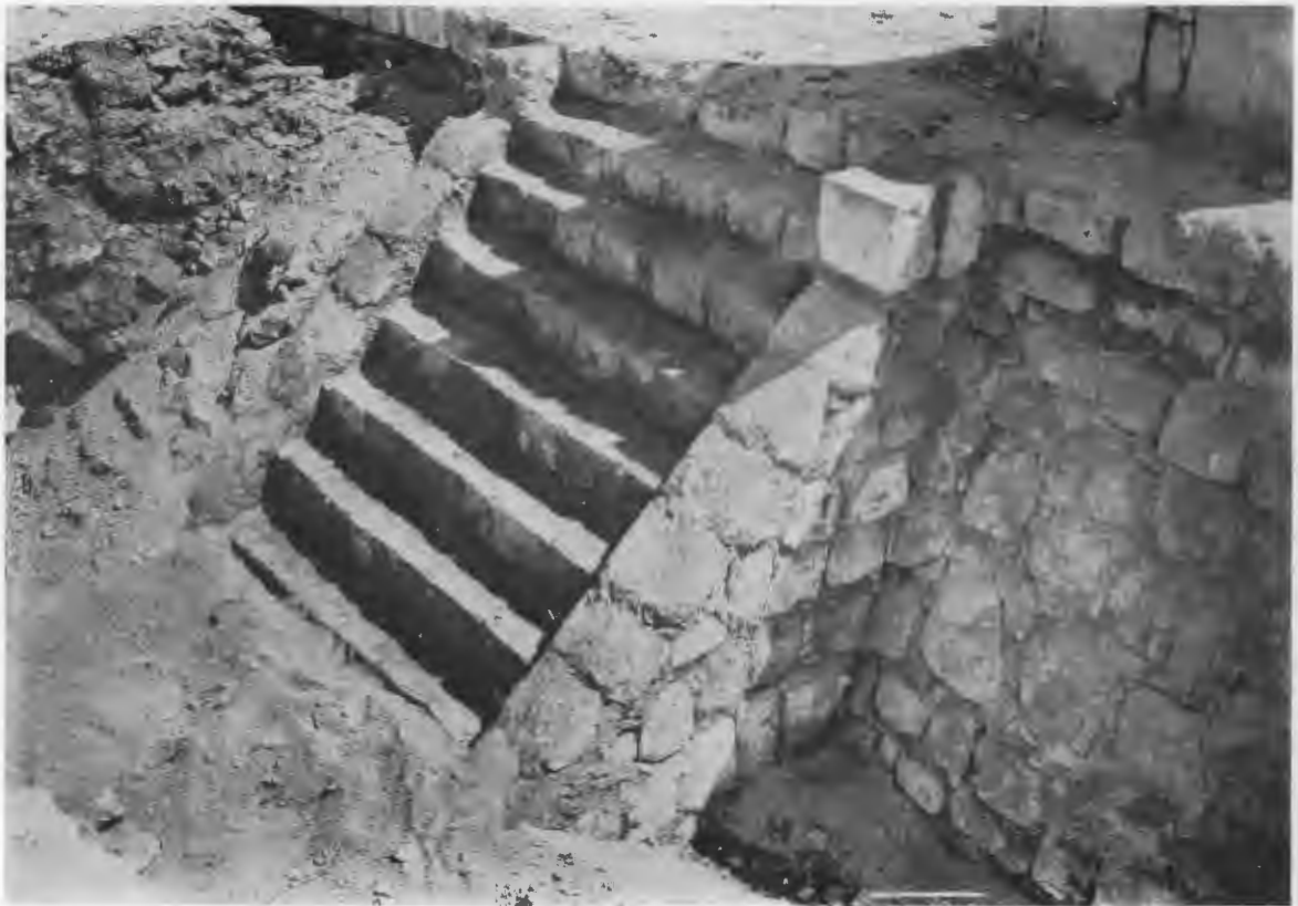
FIG. 312—CARACOL WEST ANNEX. STAIRWAY OF EARLY PLATFORM.
