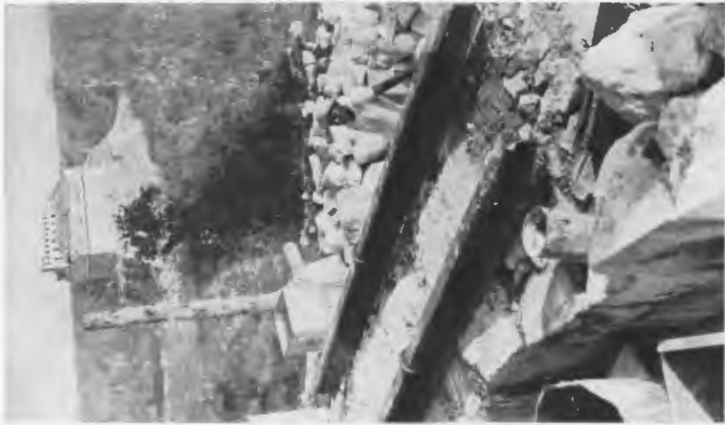
FIG. 251—Steel rails resting on top of lintel. A bolt hooked over each rail extends through holes drilled in lintel and is secured by steel plates and nuts mortised in soffit of lintel.
