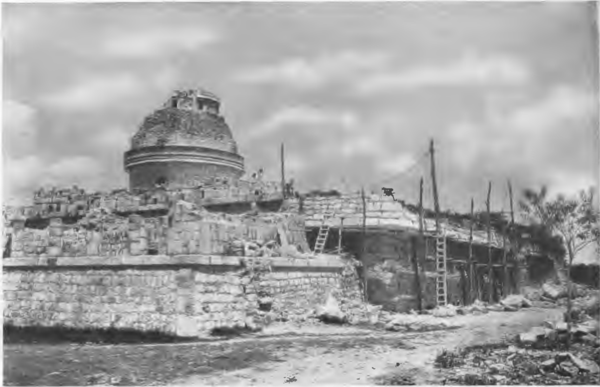
FIG. 23—LOWER PLATFORM, SOUTHWEST CORNER. REPAIRING OVERHANGING APRON MOLDING.
