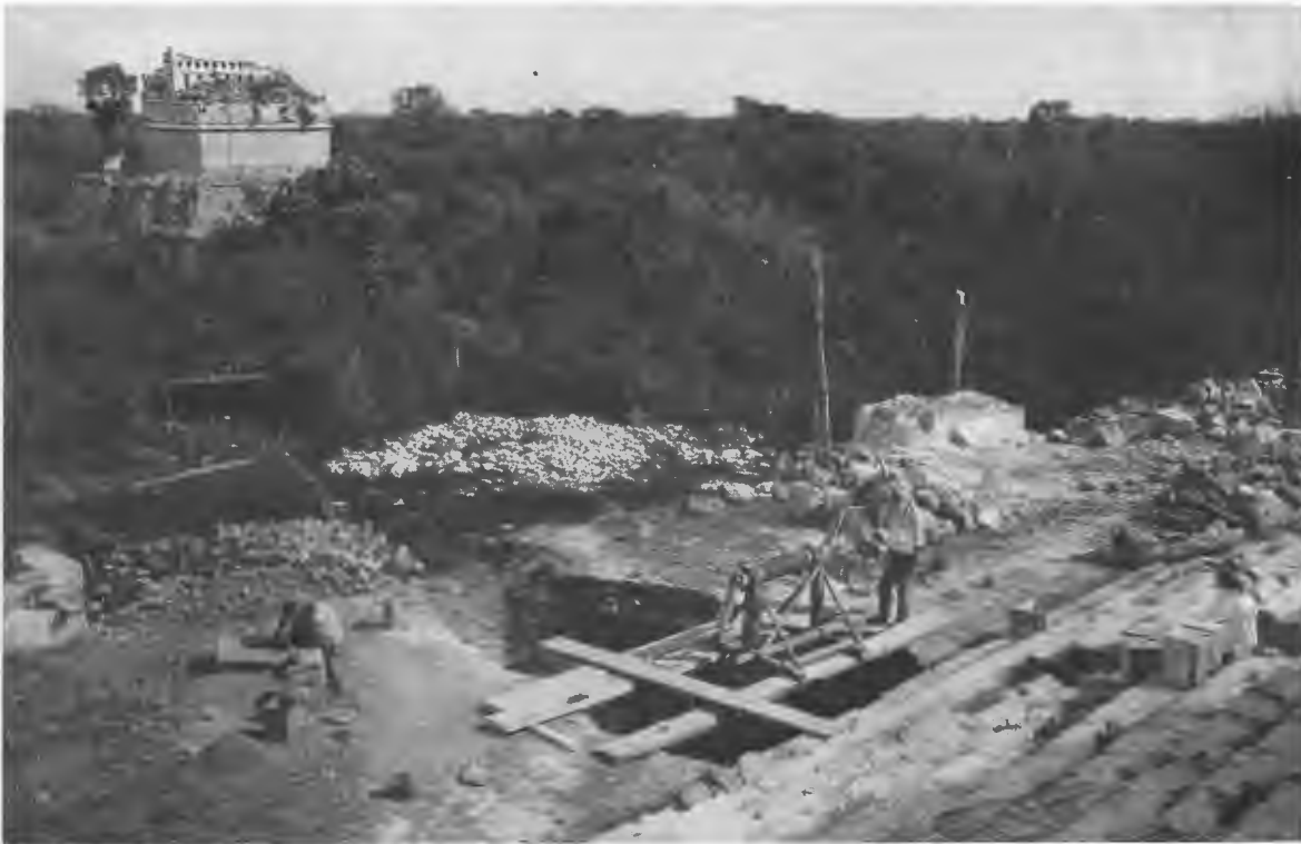
FIG. 43—WEST TRENCH, LOWER PLATFORM. A home-made winch placed on planks over trench was used to aid in removal of material.
