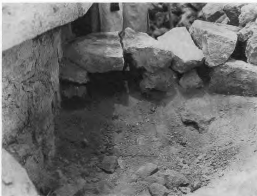
FIG. 152—MANNER OF CONSTRUCTING WEEP HOLE FROM ITS ORIFICE AT BASE OF BENCH ON NORTH SIDE, THROUGH THE Embutido SURROUNDING OUTER CIRCULAR PLATFORM.
