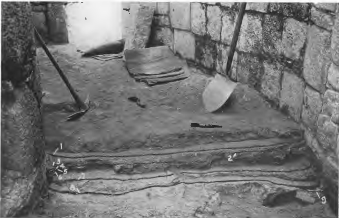
FIG. 282—FLOORS AND WORKING LEVELS SHOWN BY PAINTED BLACK LINES.
