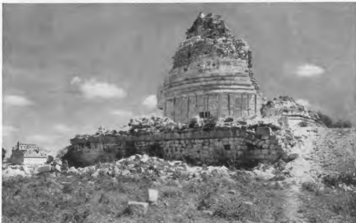
FIG. 204—PORTION OF FIVE-MEMBER MOLDING OF SOUTH SIDE REPAIRED IN 1927.
