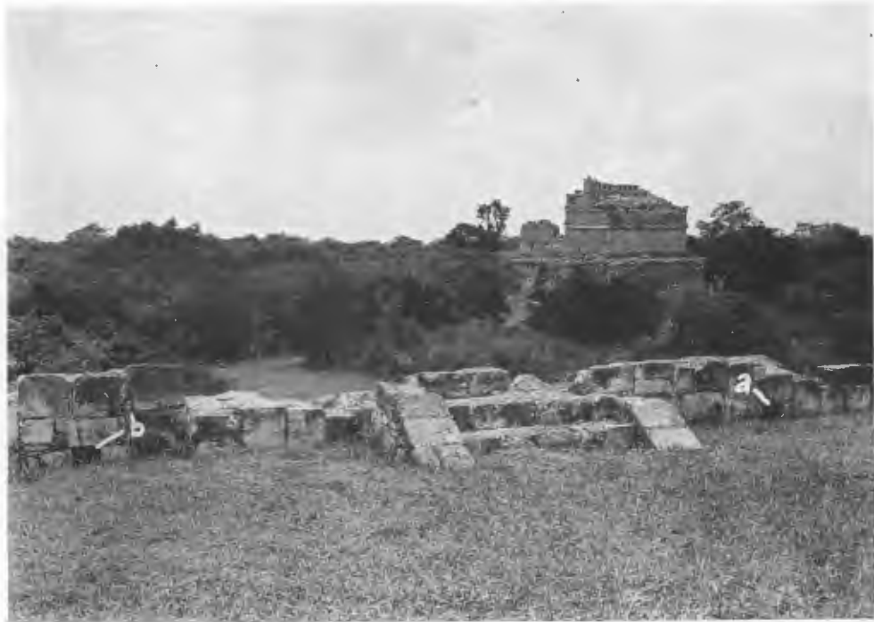
FIG. 321—STAIRWAY FROM CARACOL LOWER PLATFORM TO ROOF OF WEST ANNEX AS REPAIRED.
