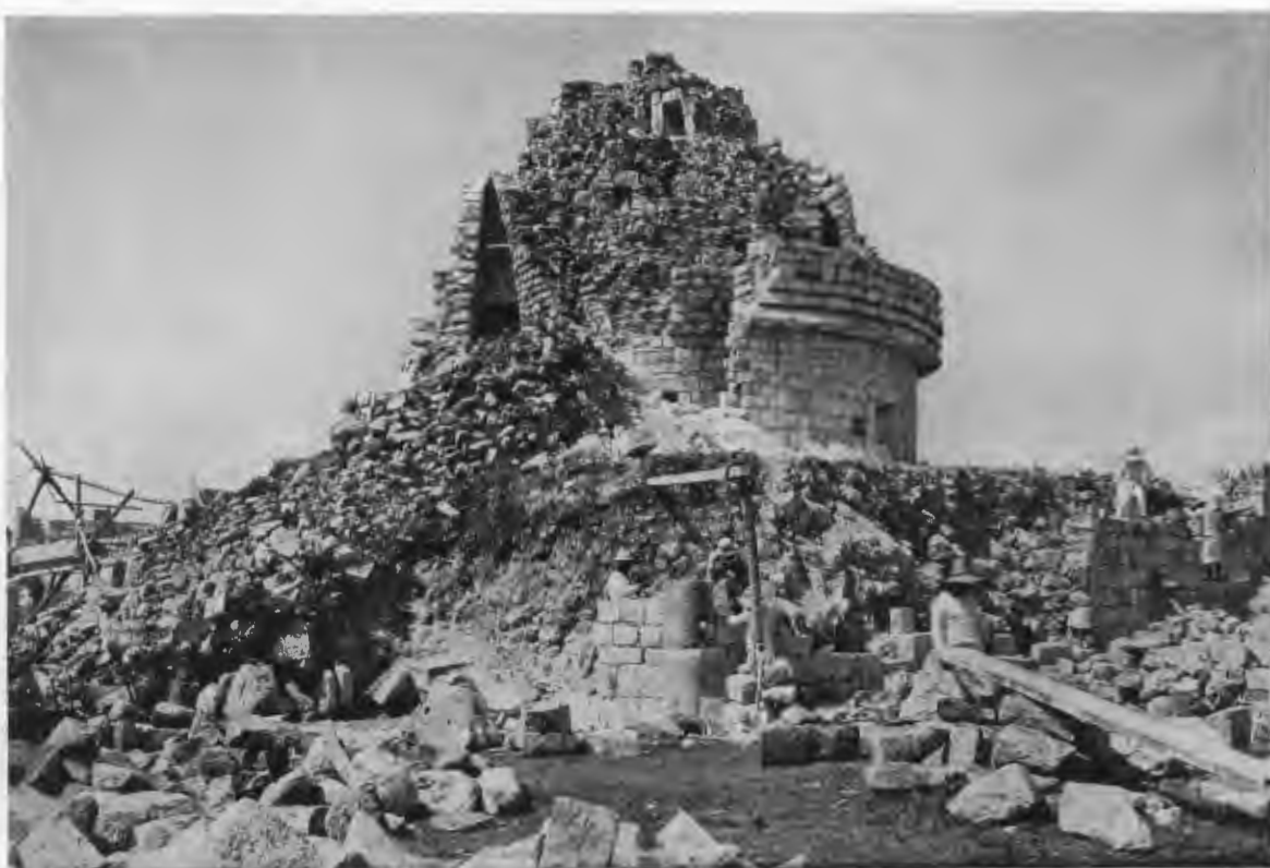
FIG. 138—REPAIR OF NORTHEAST CORNER OF UPPER PLATFORM IN 1929.
