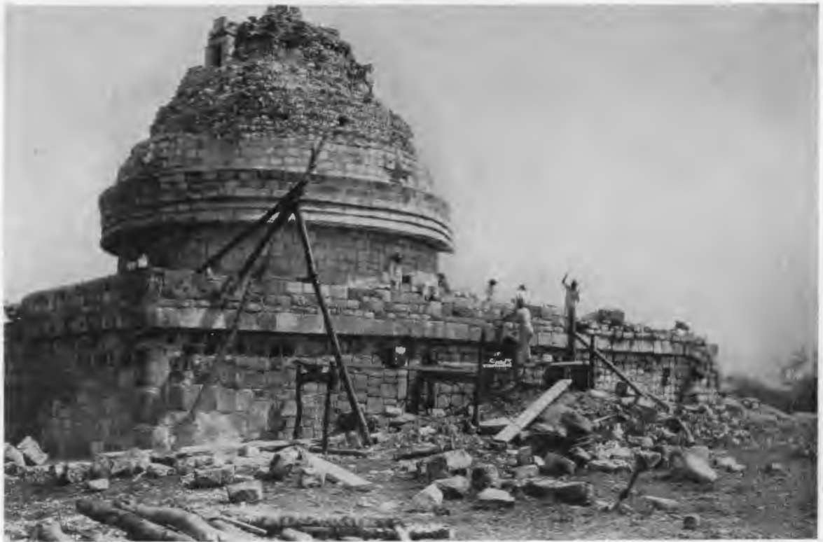
FIG. 135—UPPER PLATFORM, SOUTH SIDE, UNDER REPAIR.
