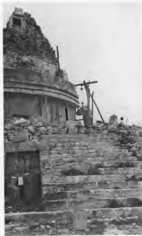
FIG. 201—SECTION OF FIVE-MEMBER MOLDING REPLACED IN 1926 IS SUPPORTED BY WOODEN UPRIGHTS.
