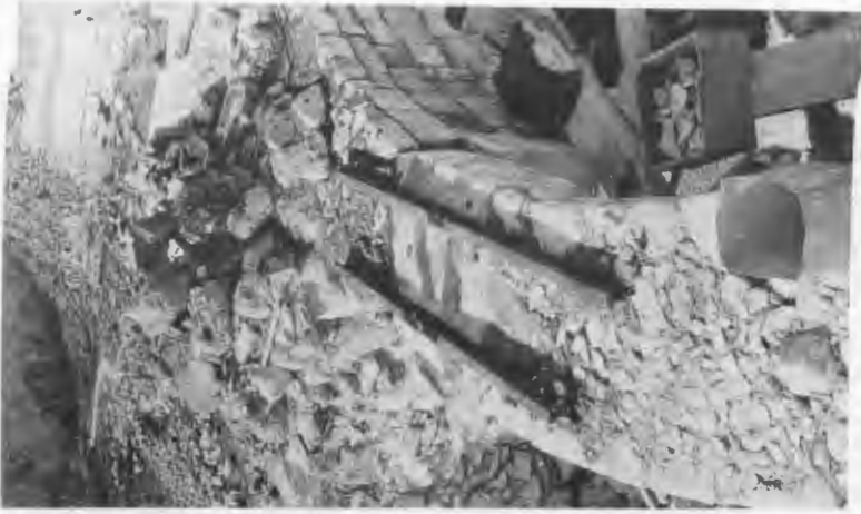
FIG. 255—Two steel rails were placed on top of lintel to give additional support to superstructure.
