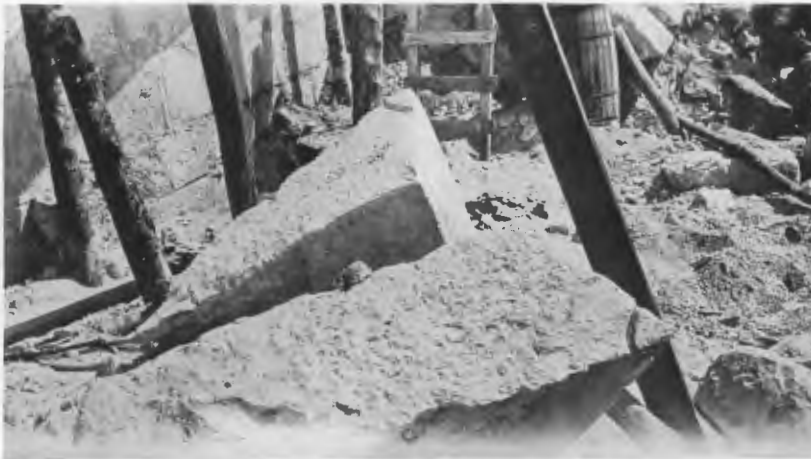
FIG. 196—CURVED GROOVE ON VERTICAL SIDE OF TWO OF THE STONES OF FIRST MEMBER OF FIVE-MEMBER MOLDING.
