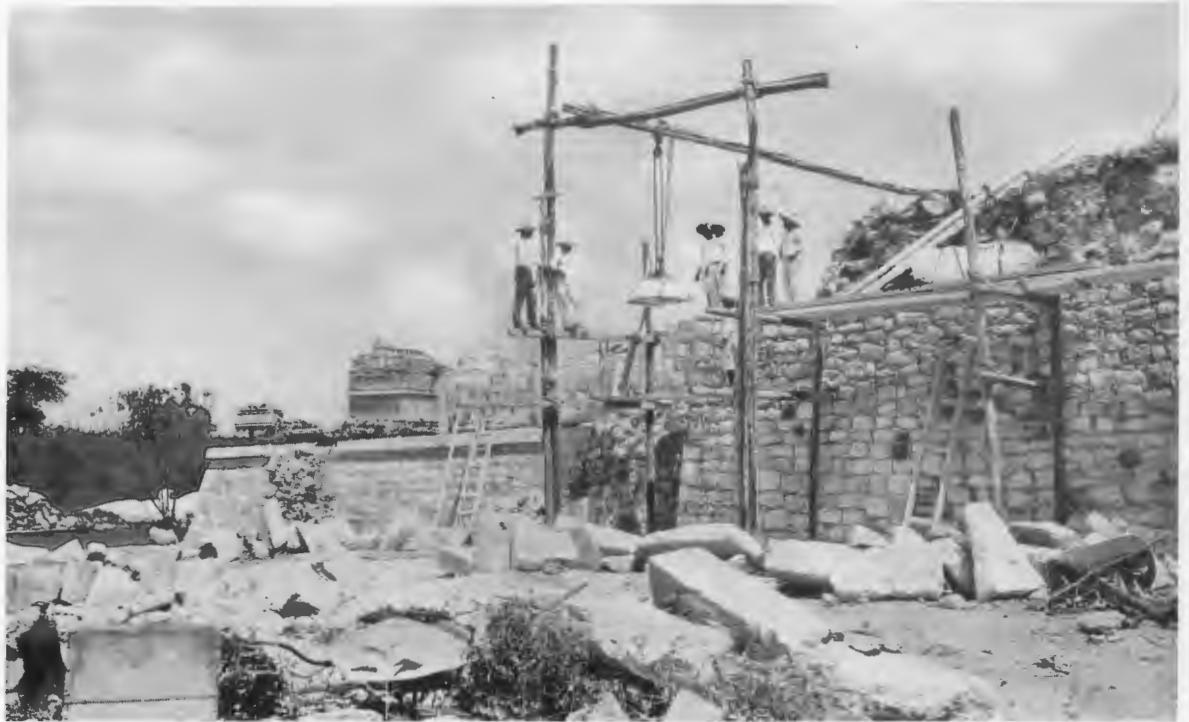
FIG. 25—RAISING BROKEN CORNER STONE OF FIRST COURSE OF OVERHANGING APRON MOLDING AT SOUTHWEST CORNER OF LOWER PLATFORM.
