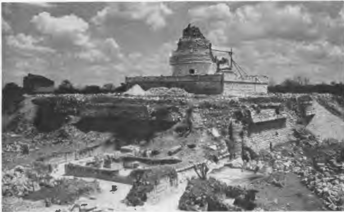
FIG. 28—LOWER PLATFORM, SOUTHEAST CORNER, BEFORE REPAIR. EAST END OF SOUTH ANNEX IN FOREGROUND.
