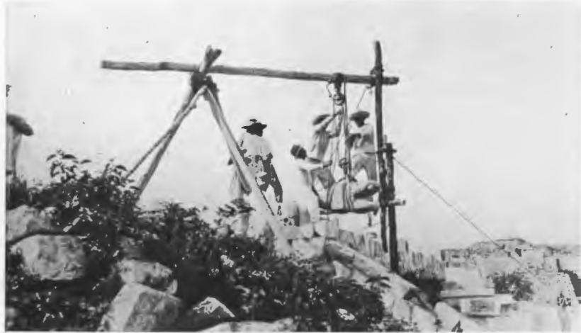
FIG. 84—REPAIR OF SOUTH BALUSTRADE OF LOWER PLATFORM STAIRWAY. Serpent head ready to swing into position.
