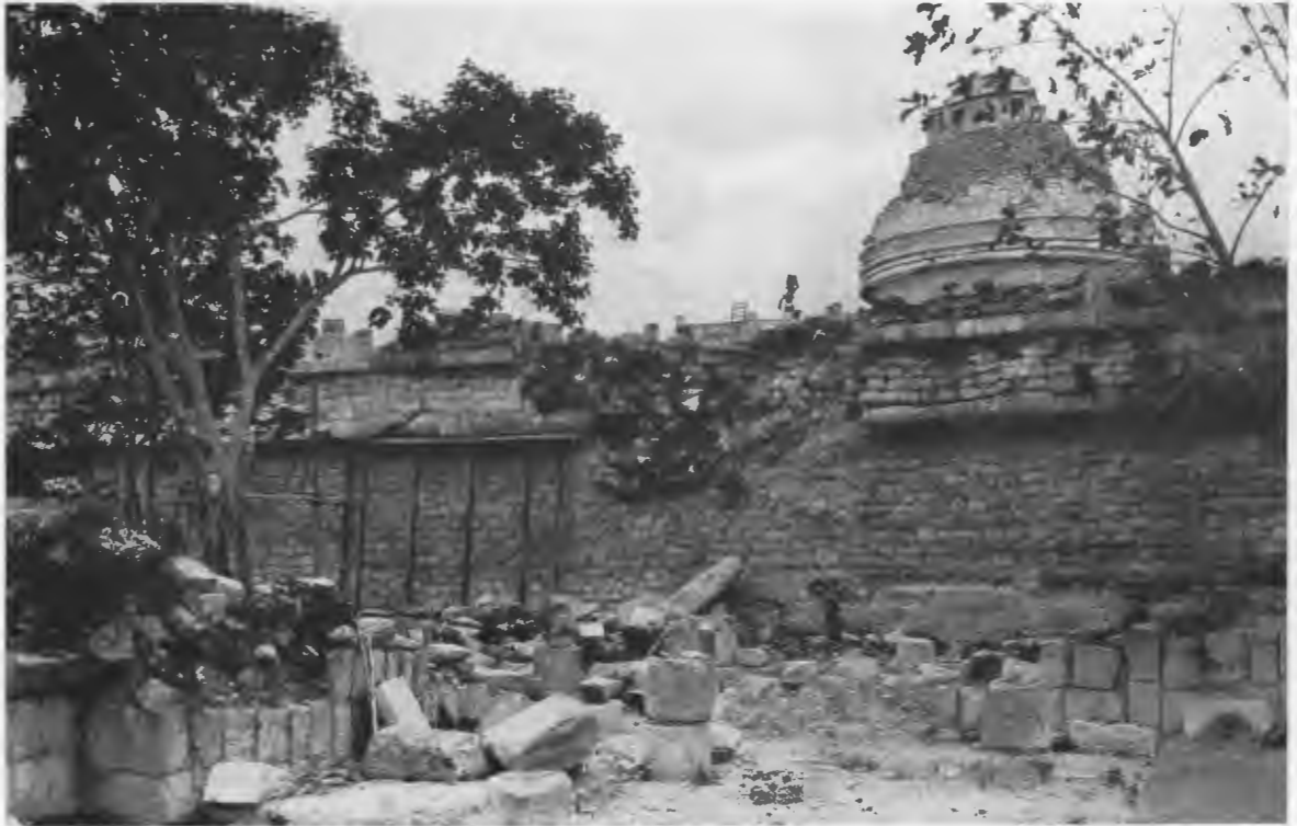
FIG. 53—LOWER PLATFORM, SOUTH SIDE. Facing of opening of passageway in apron molding has fallen.
