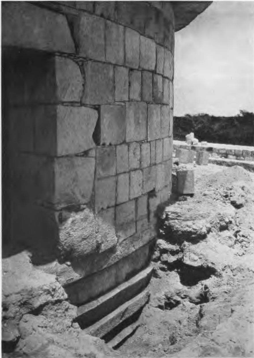
FIG. 98—SECTION OF FIRST CIRCULAR PLATFORM AS UNCOVERED NEAR EAST DOORWAY OF CARACOL TOWER.
