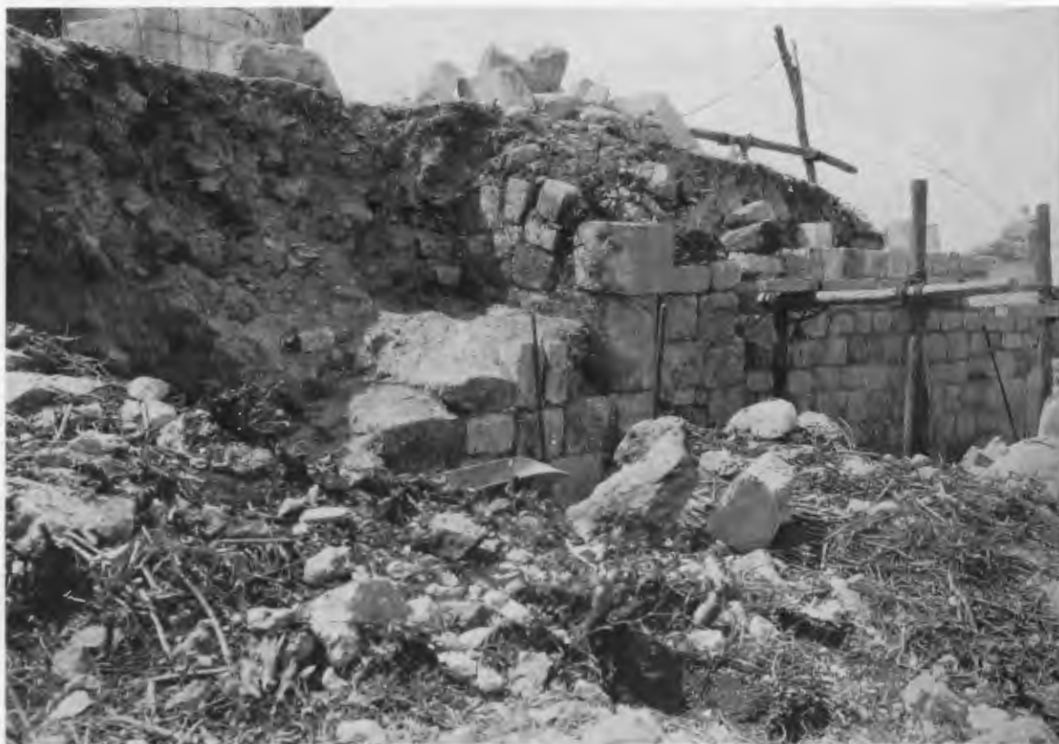
FIG. 121—NORTH SIDE OF UPPER RECTANGULAR PLATFORM. Northeast corner of first section of this platform is standing except for cornice.
