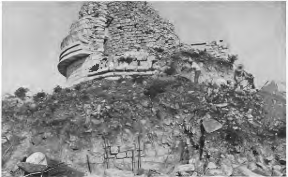
FIG. 198—CARACOL, UPPER PLATFORM AND TOWER, EAST SIDE. a , block of fallen molding.
