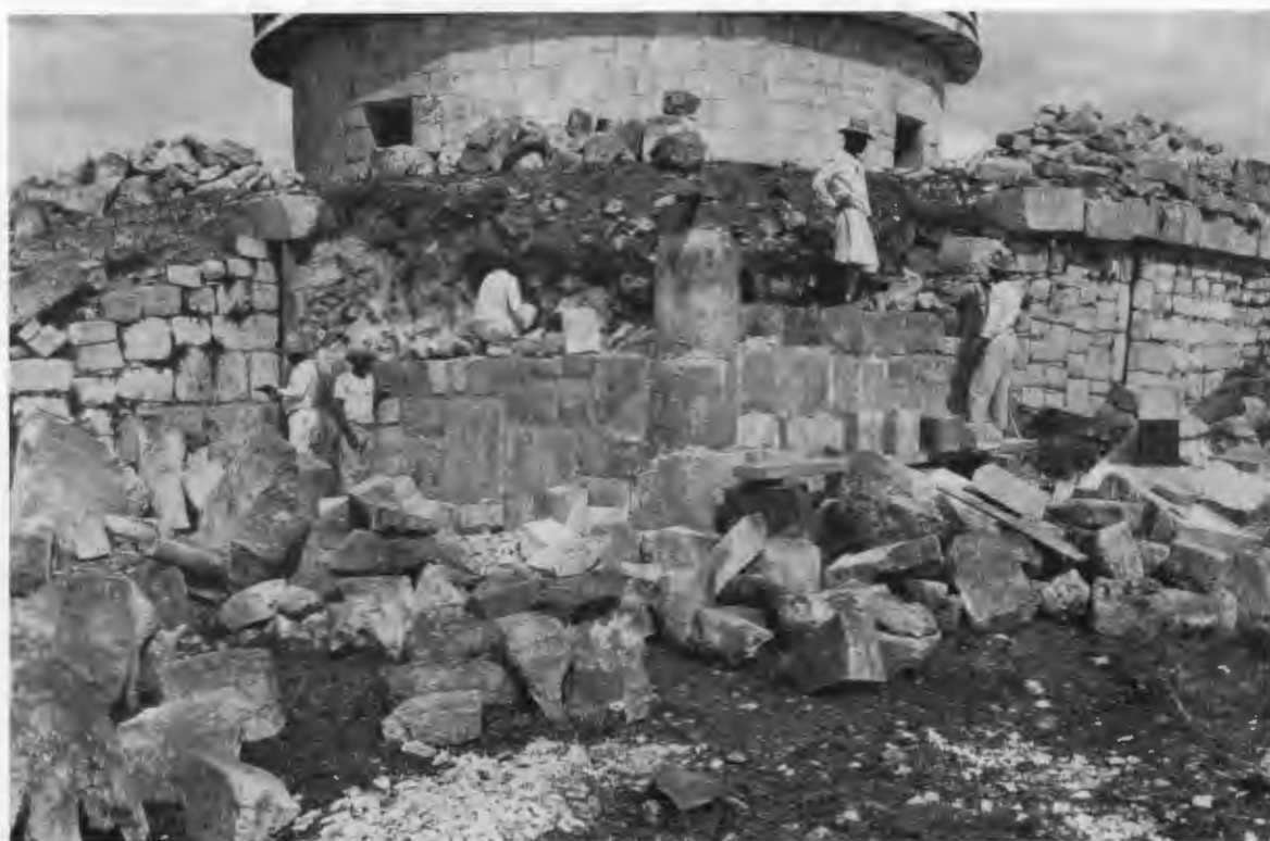
FIG. 134—SOUTHWEST CORNER OF UPPER PLATFORM UNDER REPAIR IN 1929.
