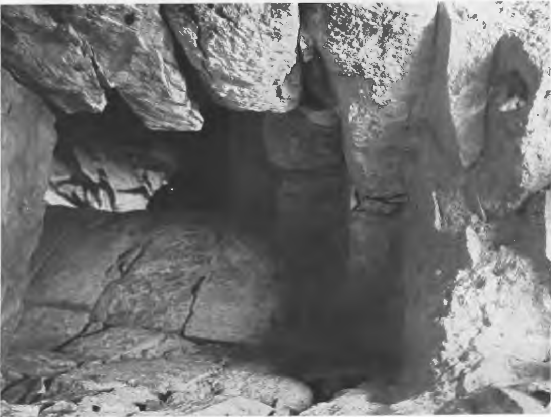
FIG. 285—CARACOL TOWER. ENTRANCE TO SPIRAL STAIRWAY IN MASONRY CORE.
