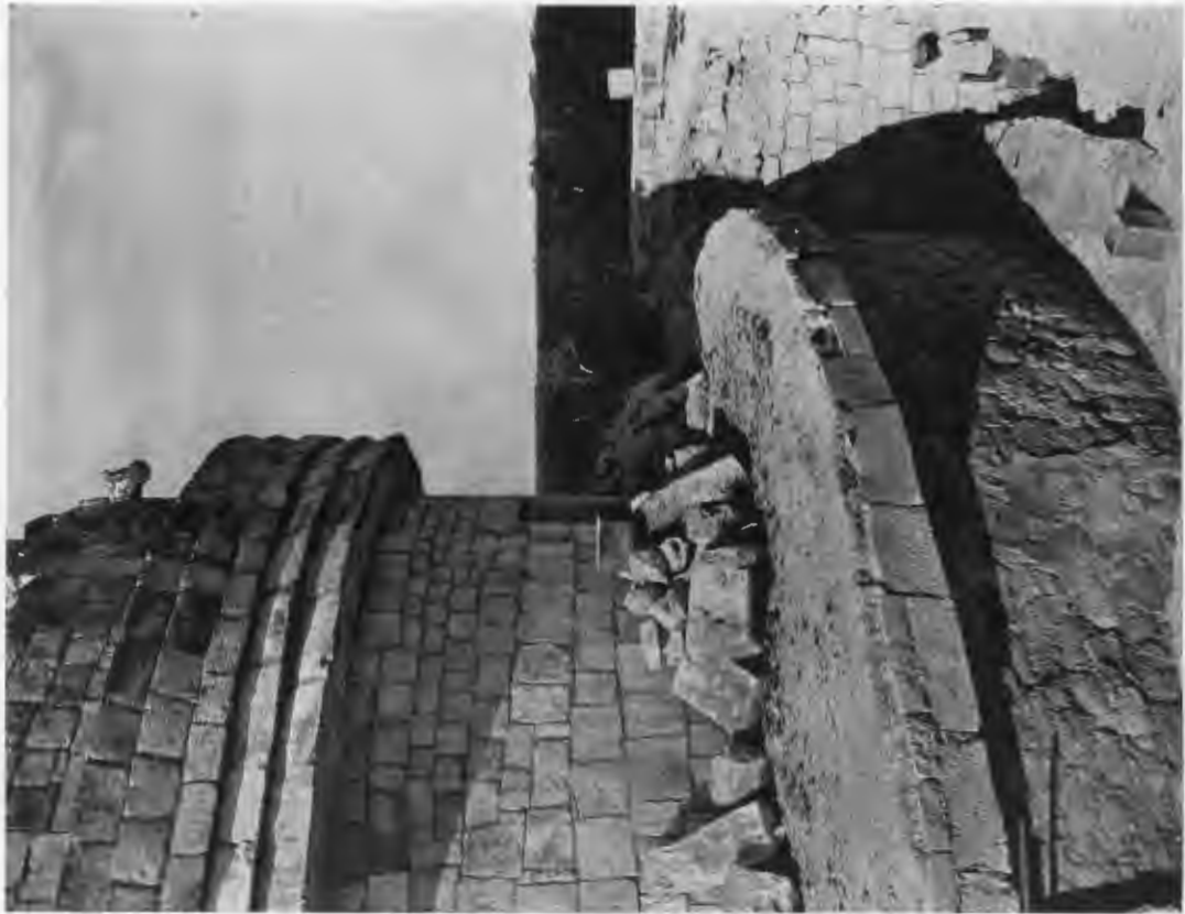
FIG. 107—SECOND CIRCULAR PLATFORM, NORTH SIDE. Man leans against north portion of east wall of rectangular platform.
