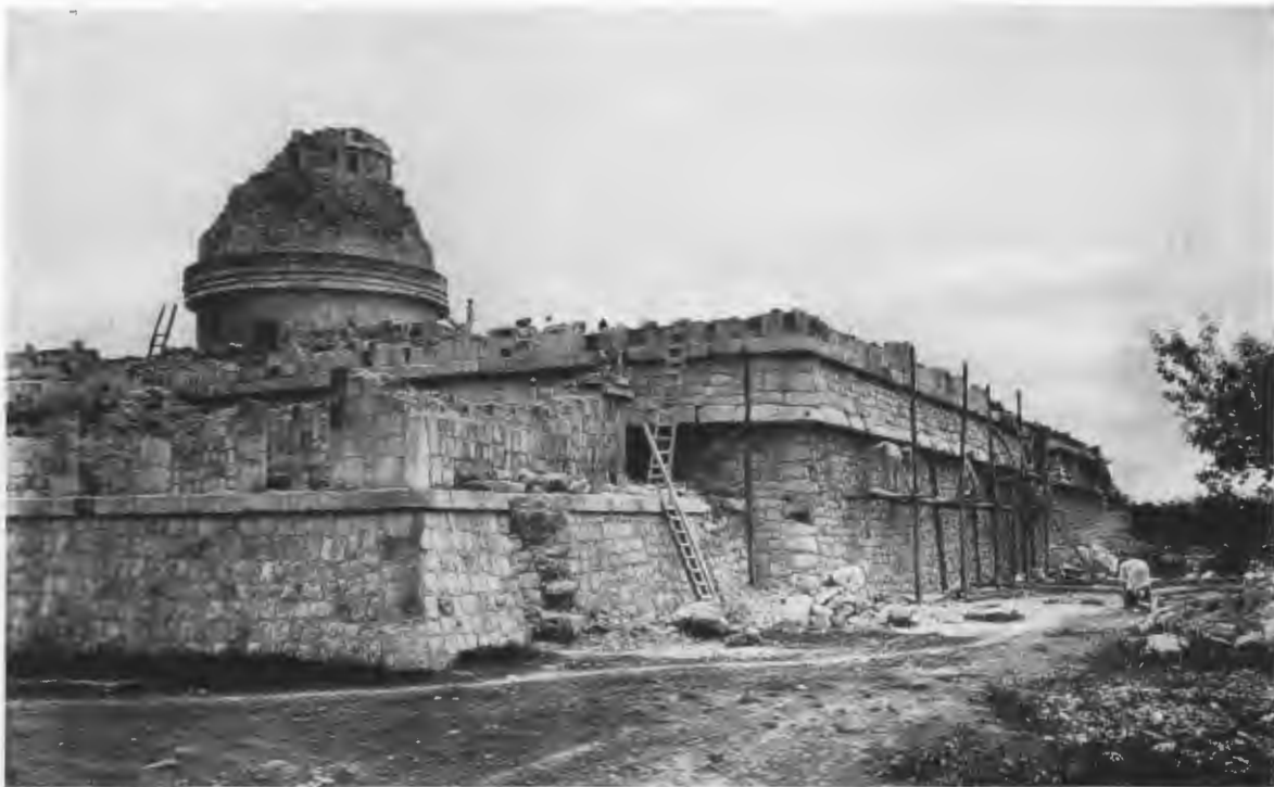
FIG. 24—REPAIR OF OVERHANGING APRON MOLDING, BAND AND PARAPET COMPLETED.
