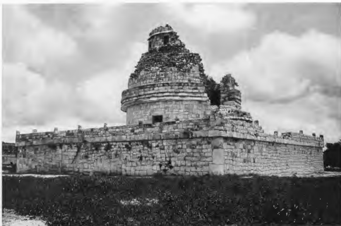
FIG. 142—UPPER PLATFORM AND TOWER. View of southeast corner taken in 1930, after repair was completed.
