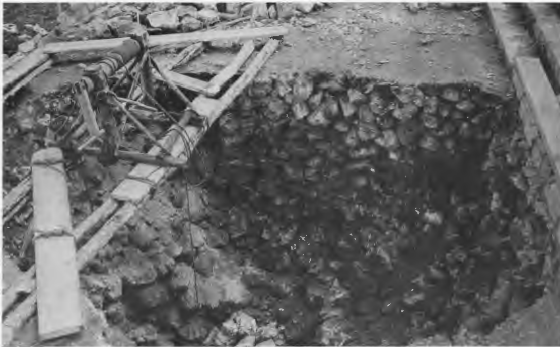
FIG. 34—WEST TRENCH, LOWER PLATFORM. Dry masonry wall extends out from under stairway. The home-made winch was used to aid in raising material to the surface.
