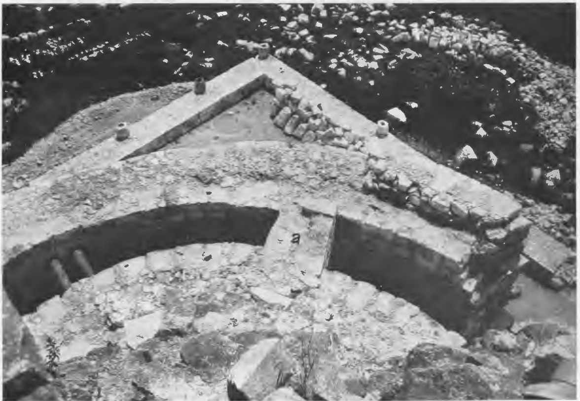
FIG. 265—INNER AND OUTER SLOPES OF ARCH IN NORTHEAST QUADRANT OF OUTER CHAMBER. Replaced to a height of 2.35 meters. The northeast buttress, a , was raised to the height to which the arch was restored.
