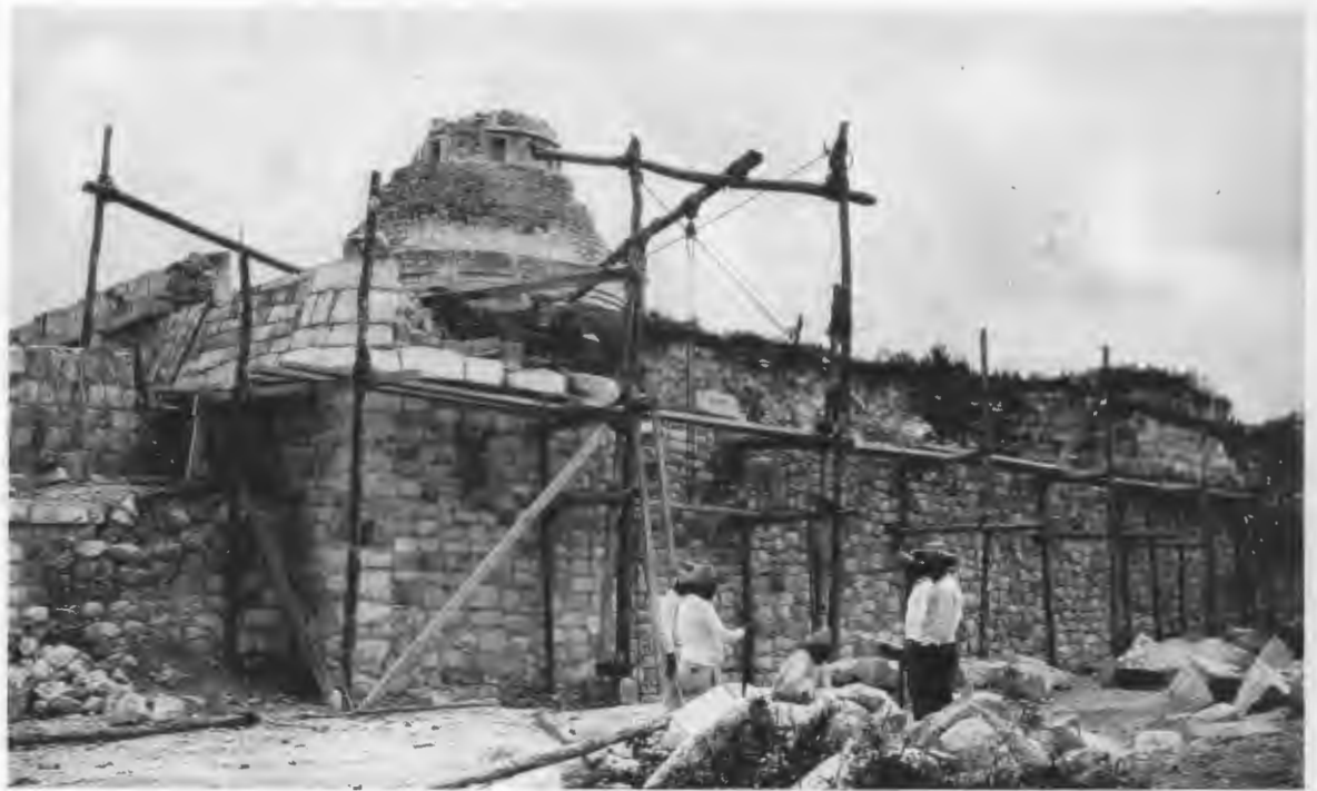
FIG. 22—REPAIRING OVERHANGING APRON MOLDING.
