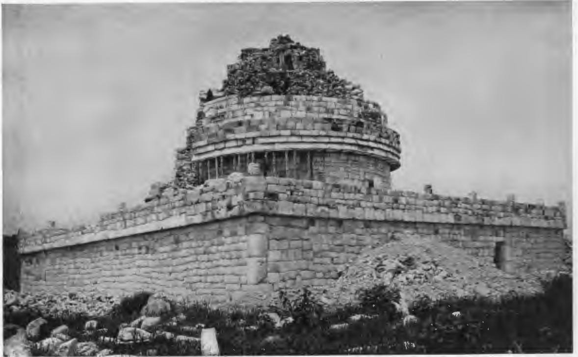
FIG. 139—NORTHEAST CORNER OF UPPER PLATFORM AND TOWER. Repair completed in 1929.
