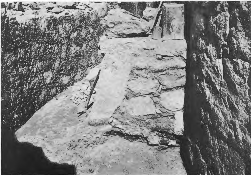
FIG. 110—END OF BENCH, NORTH SIDE OF SECOND CIRCULAR PLATFORM. A single elongated stone is used at the corner.
