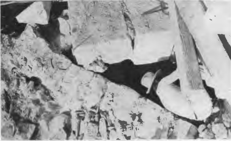
FIG. 254—Mason resetting south jamb.
