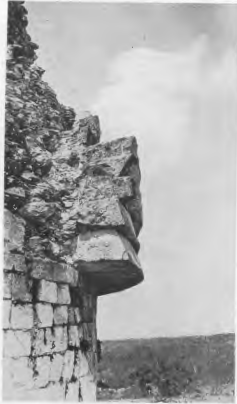
FIG. 195—SECTION OF THE FIVE-MEMBER MOLDING.
