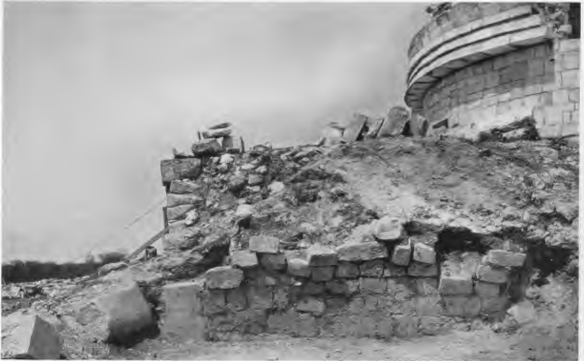
FIG. 122—EAST SIDE OF UPPER RECTANGULAR PLATFORM, SOUTHEAST CORNER.
