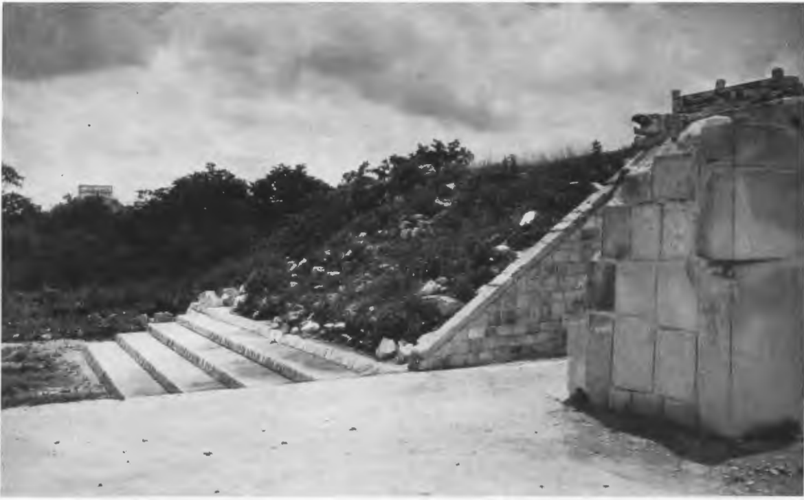
FIG. 65—FOUR STEPS, WITH BROAD TREADS, FORM LOWER SECTION OF STAIRWAY GIVING ONTO LOWER PLATFORM.
