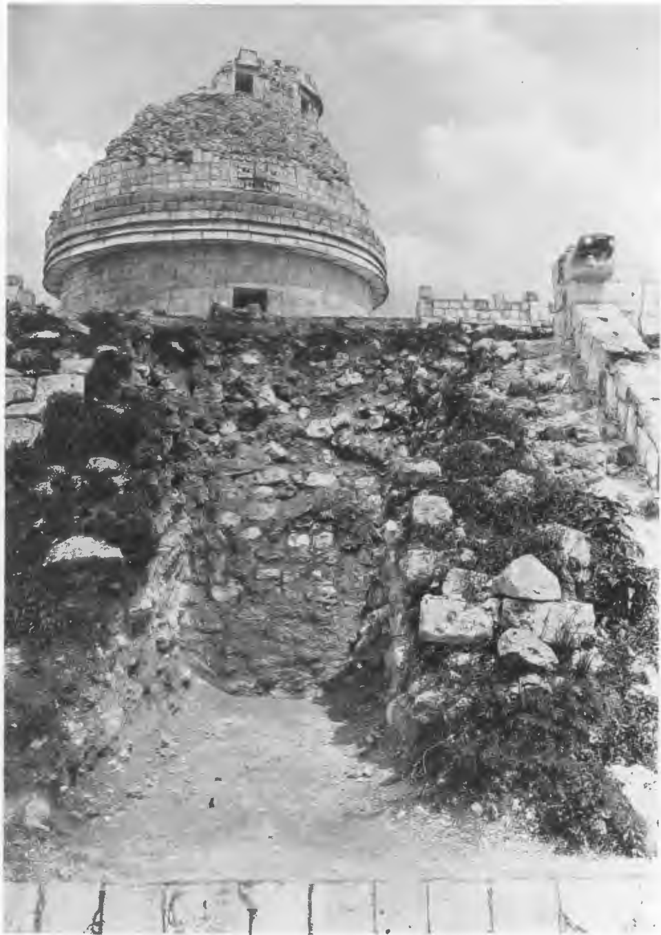
FIG. 79—STAIRWAY OF LOWER PLATFORM. Trench exposing buttress and vertical wall behind stairway.
