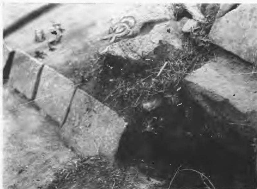
FIG. 77—LOWER PLATFORM STAIRWAY. Sculptured capping block of north balustrade found in situ .
