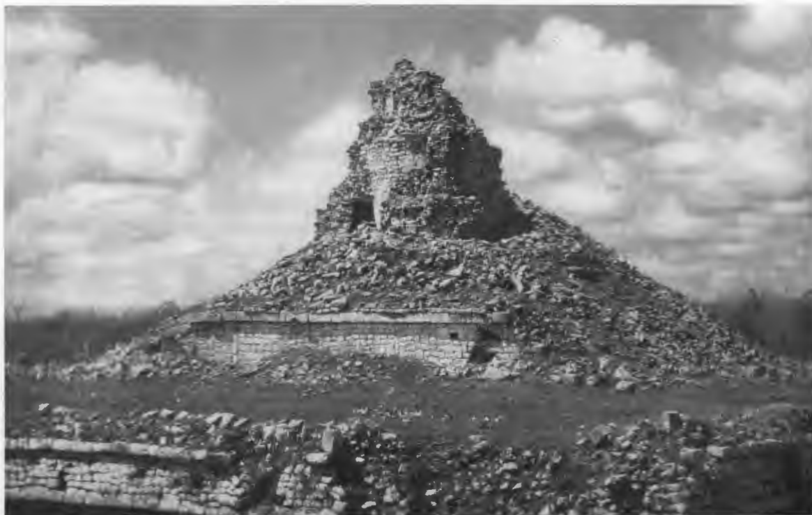
FIG. 141—UPPER PLATFORM AND TOWER. Photograph taken in 1925, showing southeast corner before repair.
