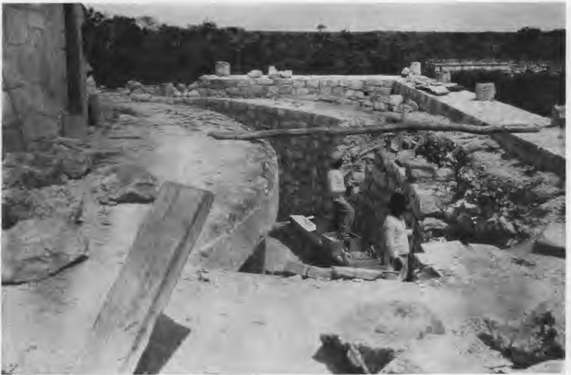
FIG. 120—MASONS WALLING OFF NORTH SECTION OF TRENCH TO LEAVE PORTION OF SECOND CIRCULAR PLATFORM EXPOSED.
