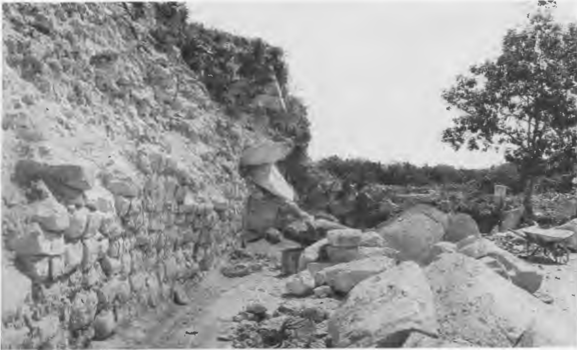
FIG. 10—LOWER PLATFORM, SOUTH SIDE. To the right are some large stones of the great apron molding recovered during excavation.
