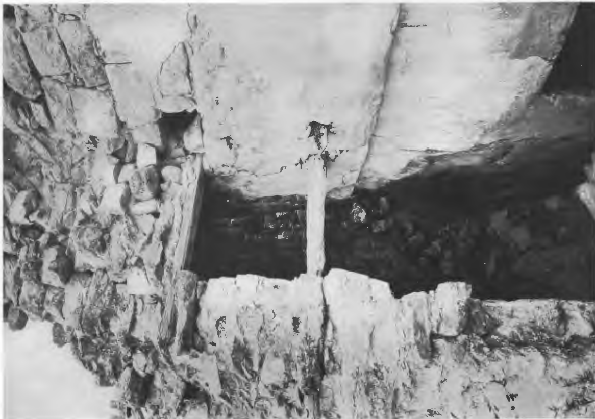
FIG. 262—Section of buttress as standing in 1925. View looking northwest.
