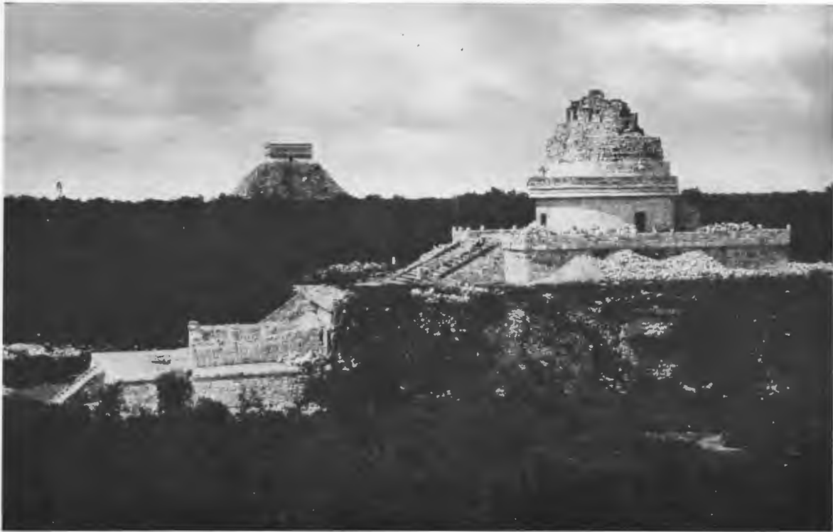
FIG. 19—CARACOL, VIEW FROM THE MONJAS. Southwest corner of lower platform before repair.
