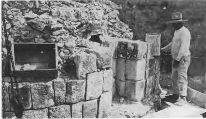
FIG. 240—CARACOL TOWER, REPAIR OF SOUTH RECESS OF UPPER STORY.
