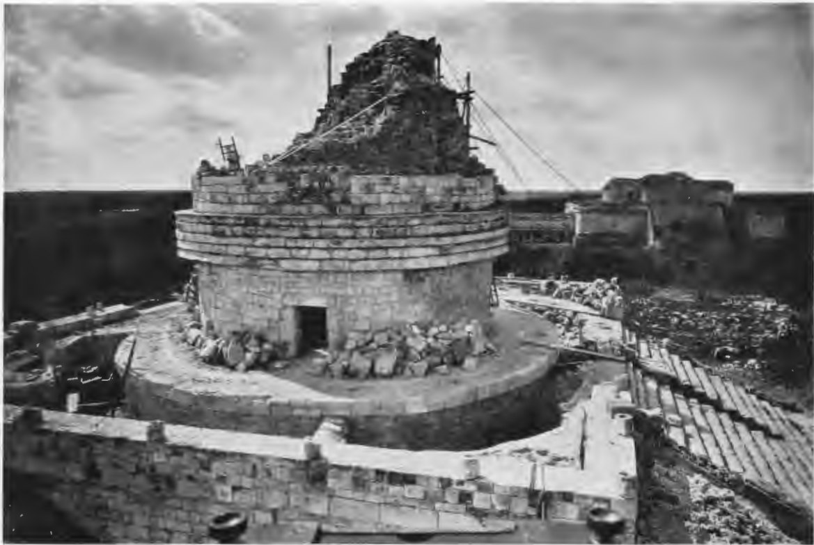
FIG. 103—VIEW OF CARACOL FROM NORTH. Second circular platform is shown enclosed by the later rectangular platform.
