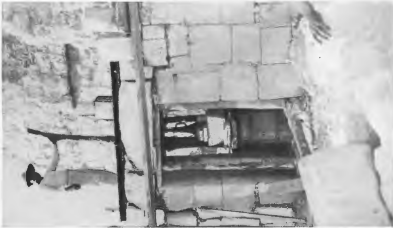
FIG. 250—Steel rails placed above lintel.
