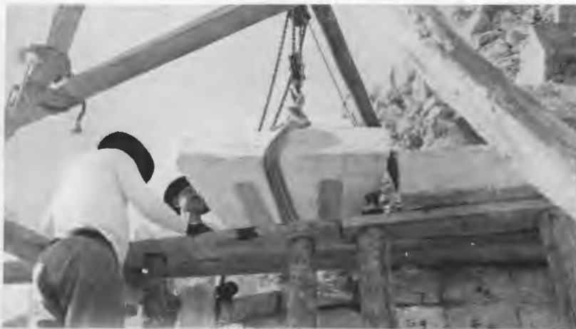
FIG. 217—MOLDING STONE, WITH GROOVES CUT ON UNDER SIDE, RAISED TO TOP OF VERTICAL WALL.
