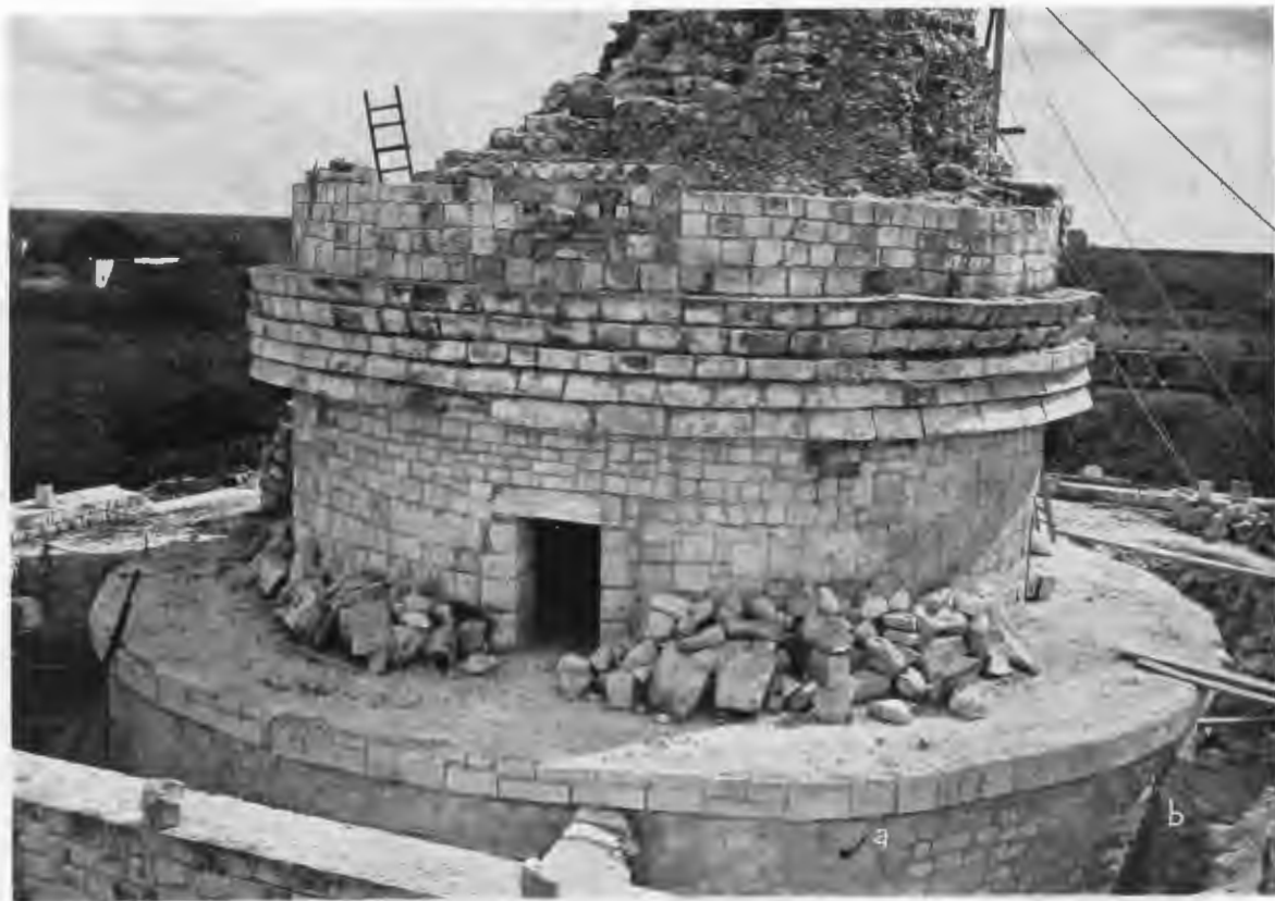
FIG. 104—VIEW OF CARACOL TOWER AND SECOND CIRCULAR PLATFORM FROM NORTH. a , orifice of weep hole; b , roughly laid wall dividing embutido of western section of rectangular platform in two tasks.
