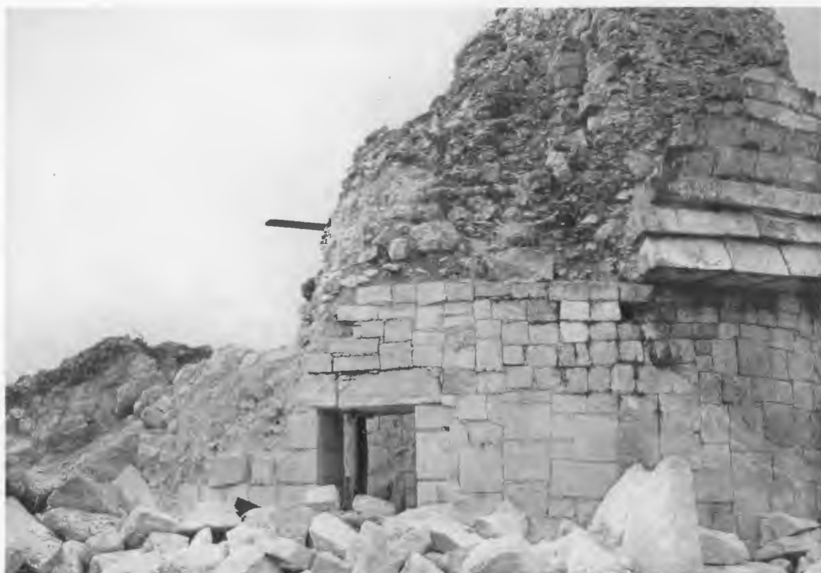
FIG. 247—NORTH DOORWAY, OUTER ANNULAR CHAMBER. THE LINTEL WAS FOUND BROKEN.
