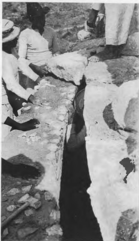
FIG. 270—MASONS CLOSING SOUTHERN SECTION OF ARCH OF OUTER ANNULAR CHAMBER.
