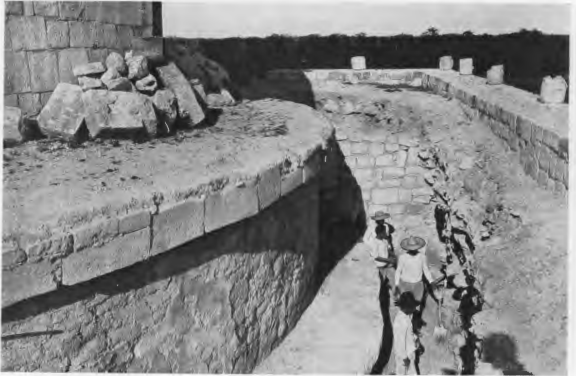
FIG. 119—EXCAVATION OF NORTH SIDE OF SECOND CIRCULAR PLATFORM.
