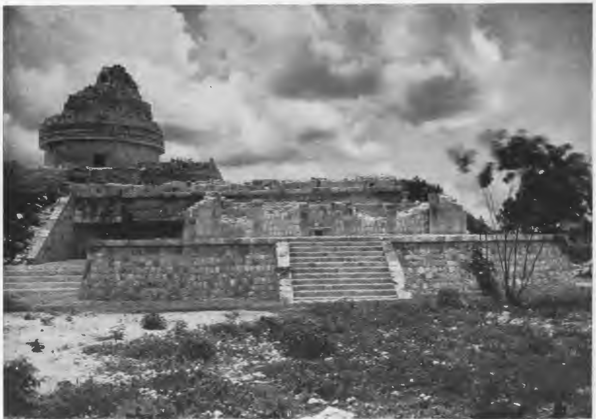
FIG. 304—CARACOL WEST ANNEX, VIEWED FROM WEST, REPAIR COMPLETED.
