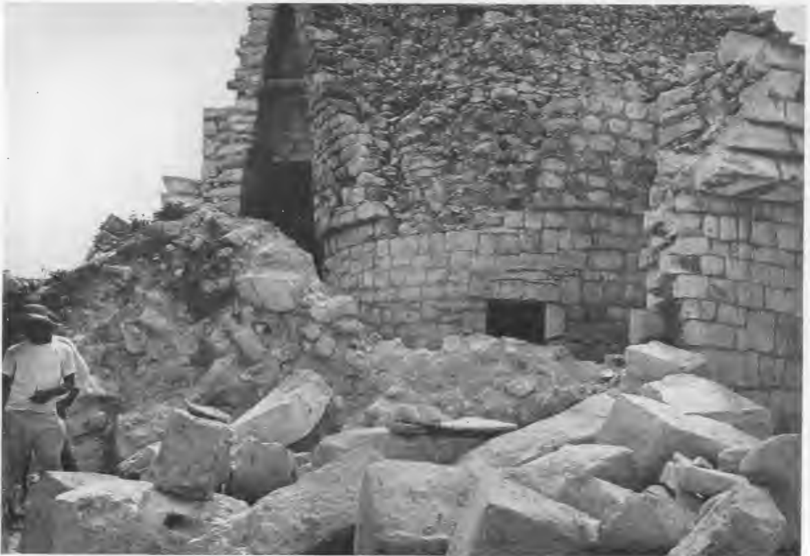
FIG. 264—NORTHEAST DOORWAY OF INNER ANNULAR CHAMBER. SOUTHEAST BUTTRESS HAS BEEN REPAIRED.
