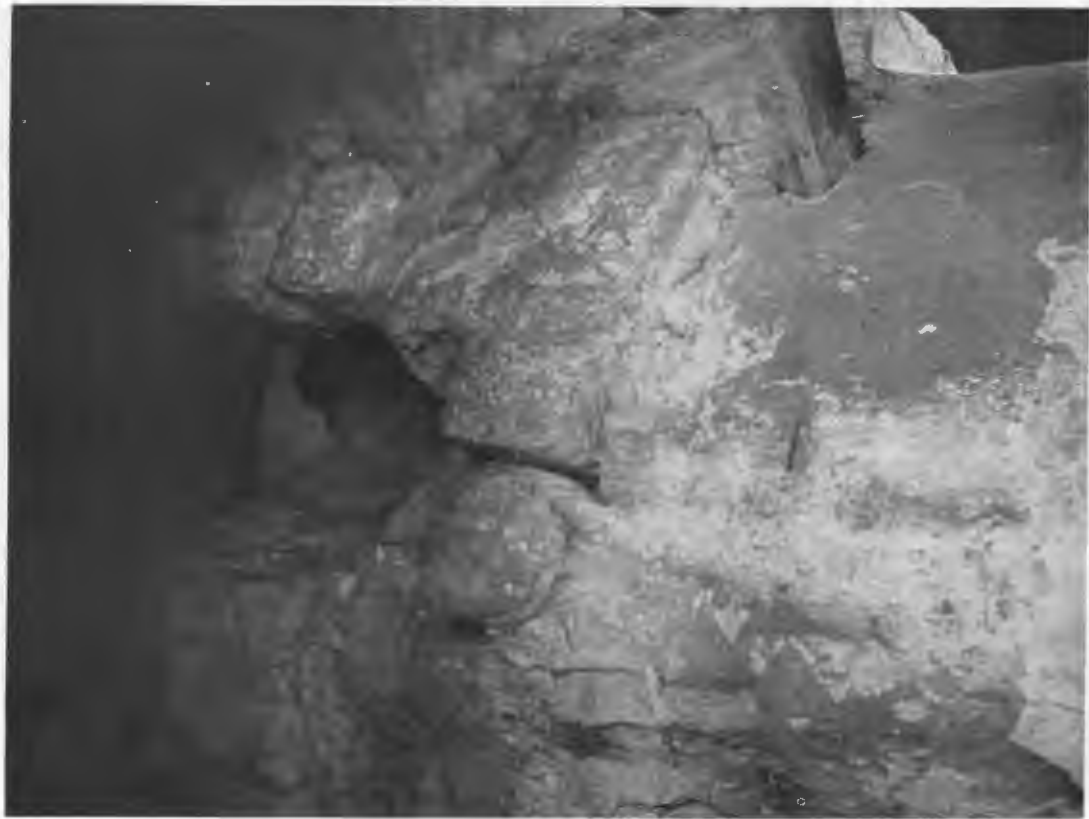
FIG. 283—OPENING IN MASONRY CORE GIVING INTO SPIRAL PASSAGEWAY.
