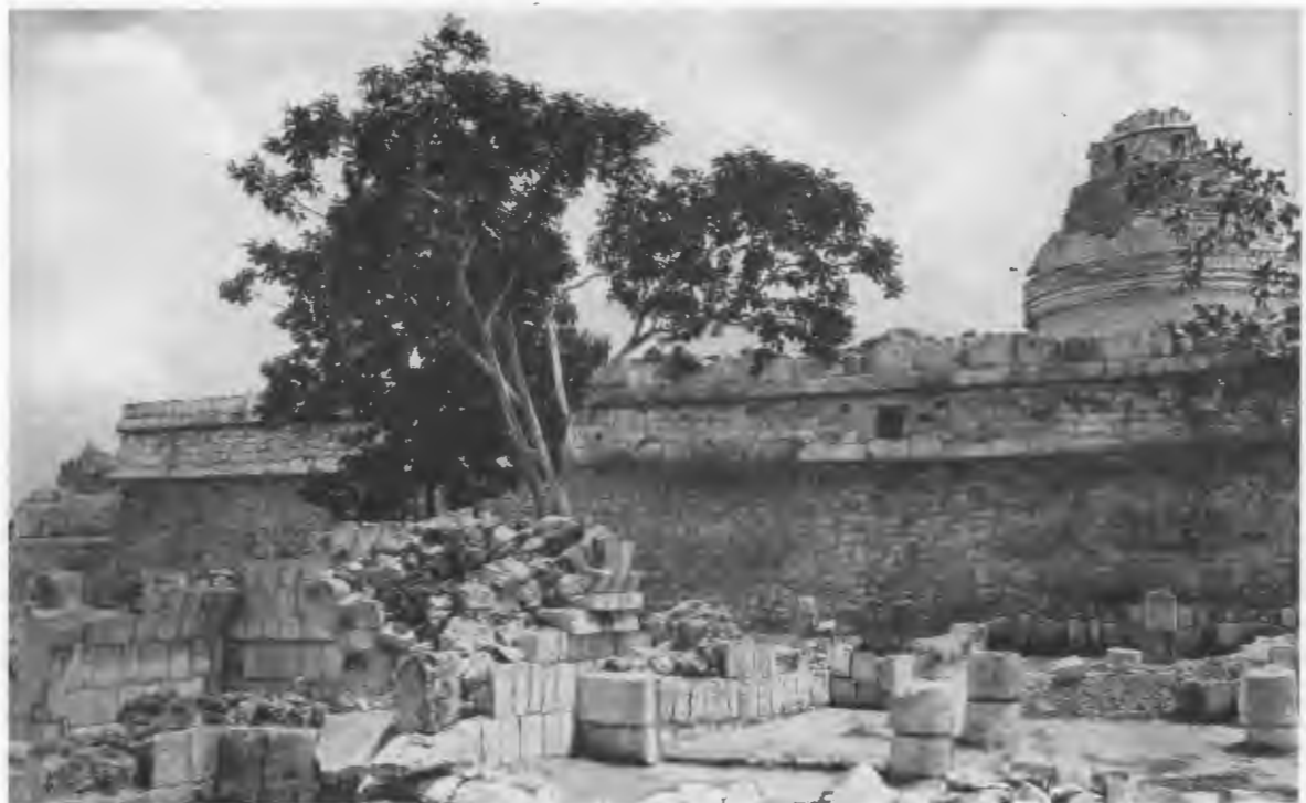
FIG. 54—LOWER PLATFORM, SOUTH SIDE. Platform facing and opening of passageway repaired.
