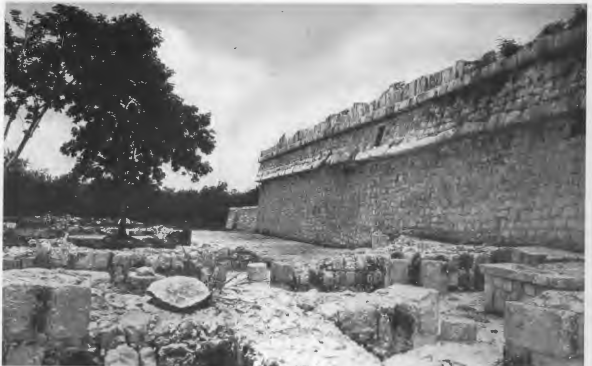
FIG. 26—SOUTH SIDE OF LOWER PLATFORM, LOOKING TOWARD SOUTHWEST CORNER. REPAIR COMPLETED.
